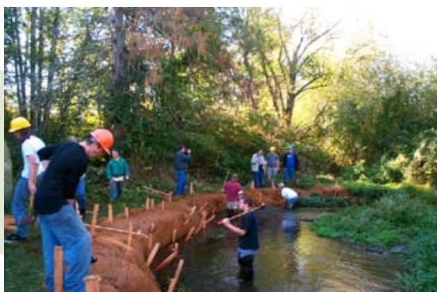
Construction of the brush mattress underway.
