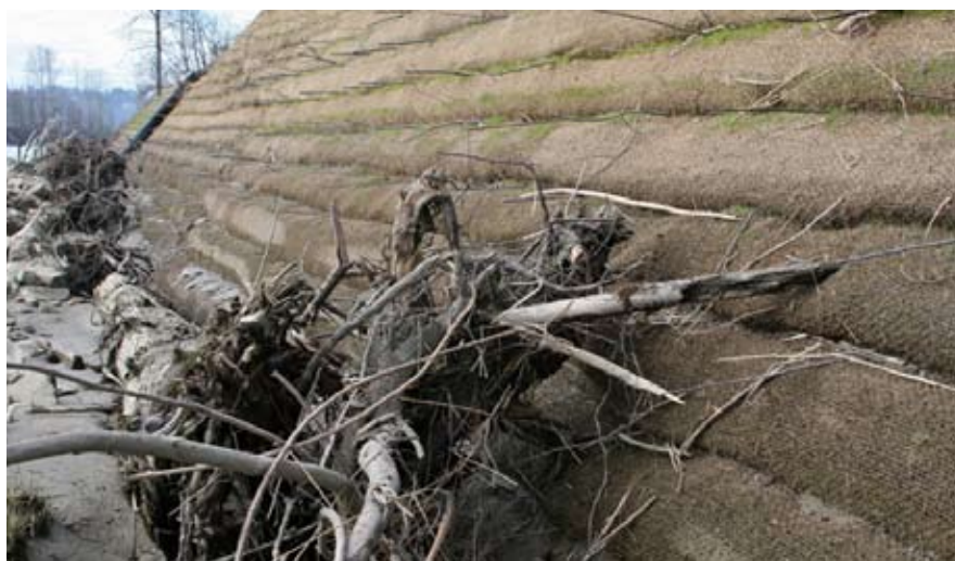
The offsetting of the soil wraps comprising the structural earth wall (SEW) give it its step-like appearance. The logs anchored to the toe of the embankment protect the structure from fast flowing woody debris and provide habitat for migrating fish during high water.
