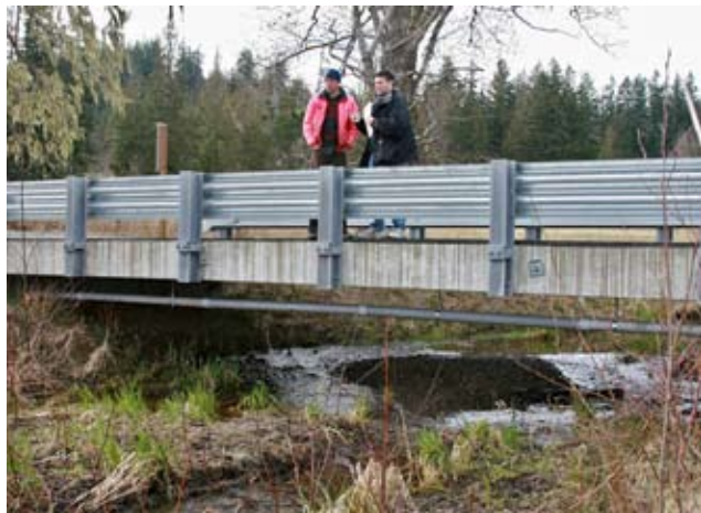
The extra wide design of the bridge ensures adequate room for water flow during flood conditions.
