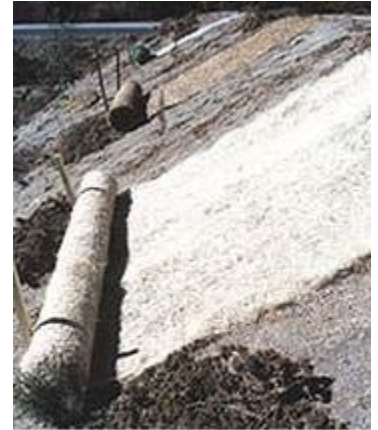
Several types of erosion control blankets are in the process of being installed on a slope to evaluate their effectiveness.
