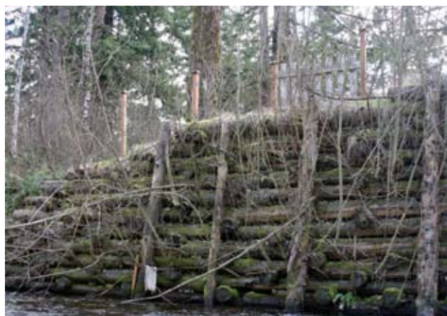
The crib wall will overgrow with vegetation, which will ultimately become the structure itself when the logs finally decay.
