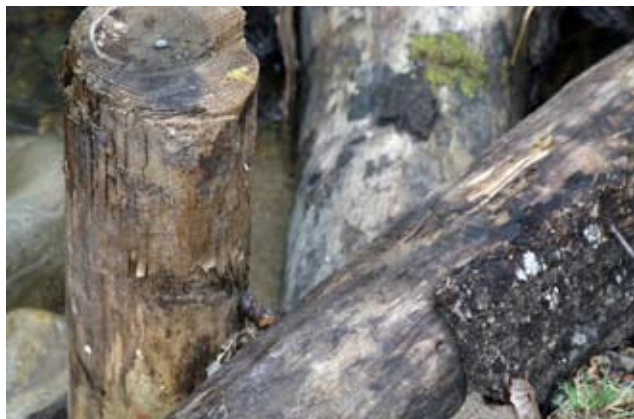
The logs in the jams are secured to each other with rebar.
