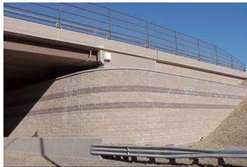
Figure 22: Founders/Meadows GRS bridge abutment.
