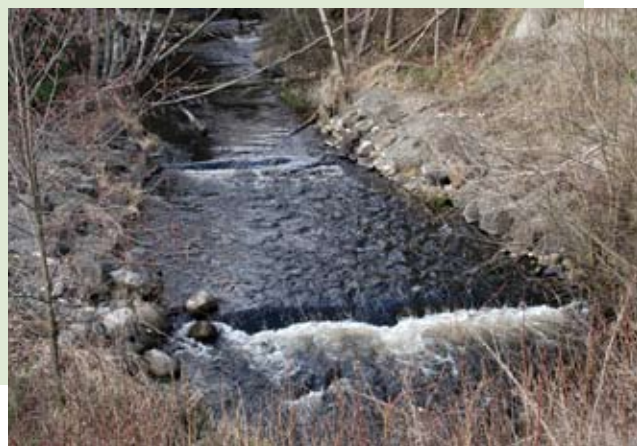
The restructured channel is now far easier for fish to traverse during migration.
