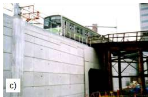
Figure 7: GRS RW having a FHR facing supporting one of the busiest rapid transits in Japan (Yamanote Line), near Shinjuku station, Tokyo (constructed during 1995 – 2000): a) typical cross-section; b) wall under construction; and c) completed wall
