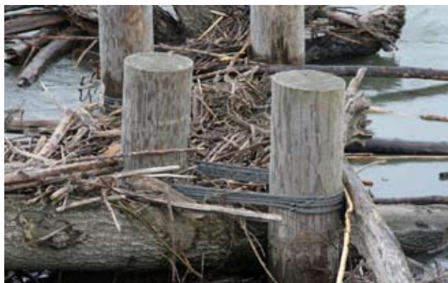
The timber piling structures capture woody debris, which provides roughness to the river, and ultimately establishes additional habitat.
