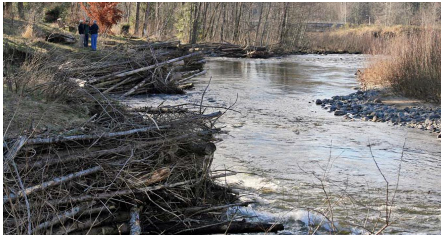
Figure 4. Logjams installed in Washington State (image from “Engineering With Nature – Alternative Techniques to Riprap Bank Stabilization,” FEMA; included in Attachment B).
