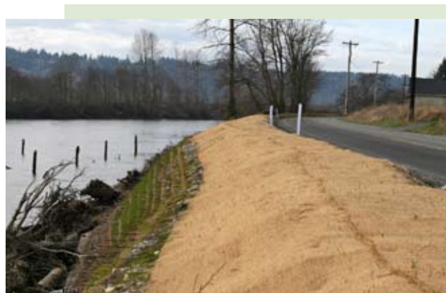
Eventually the coir fabric and the structural earth wall itself will be completely overgrown with hydro-seeded grass and other vegetation.
