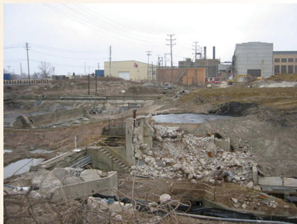
Demolition of existing infrastructure and buildings
