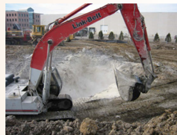
Sediment stabilization mixing operation
