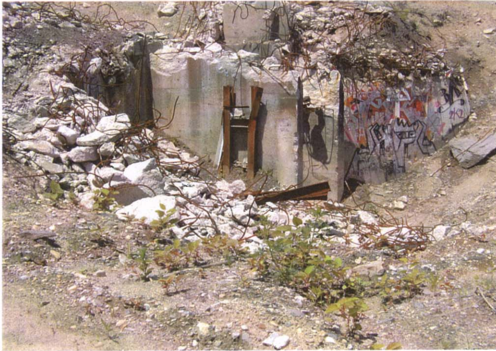
Photo 1: Remnants of the reinforced concrete material crusher foundation.
