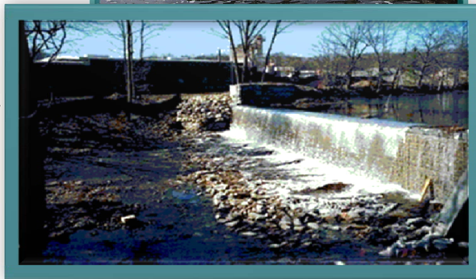
Restored Allendale Dam
