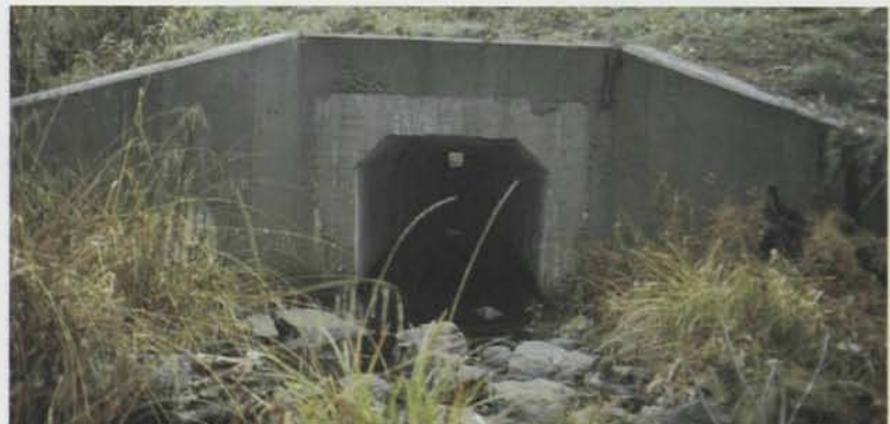
Concrete animal tunnel
