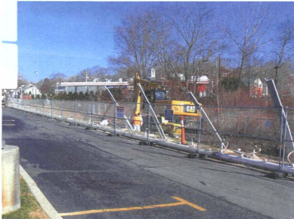
Description: Trench excavation Name: 11Dec2010 001
