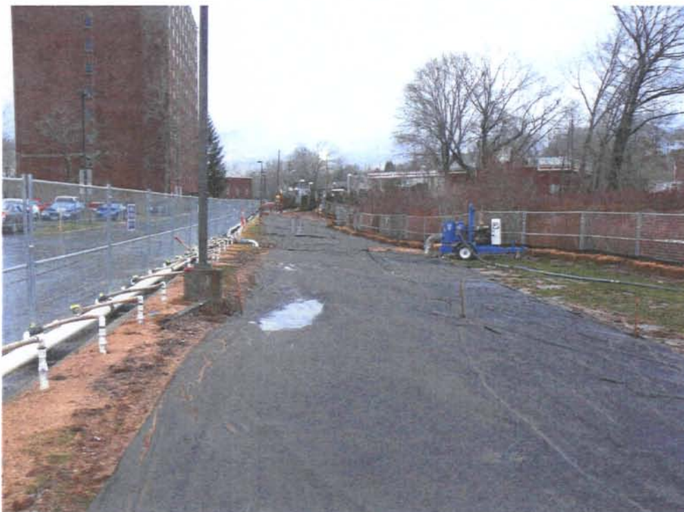
Description: Fabric over completed trench after rain Name: 13Dec2010 003
