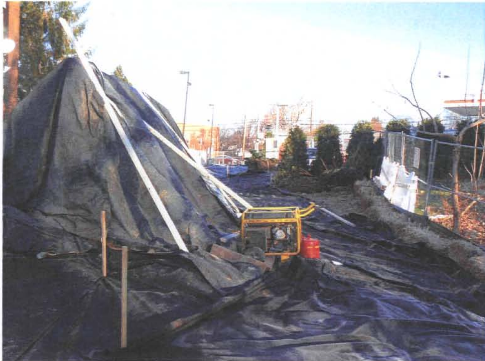
Description: "Hot Box" construction Name: 17Dec2010 017
