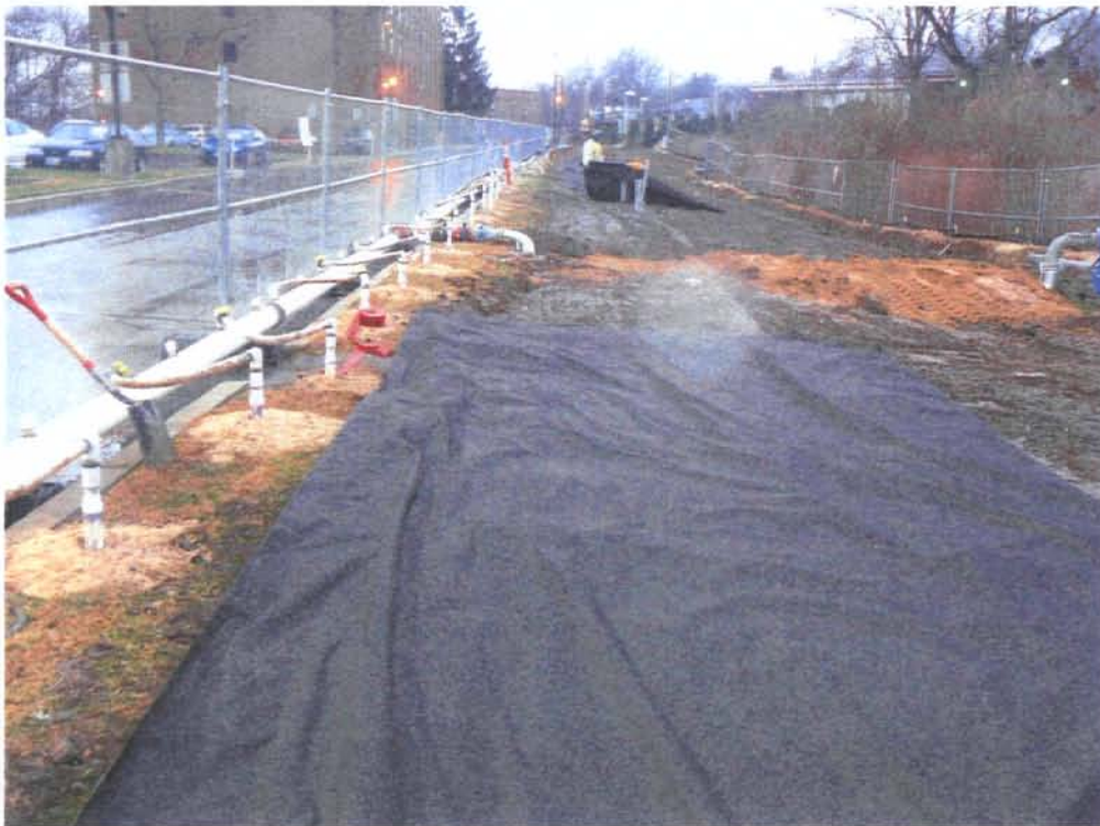
Description: Laying of fabric in preparation for rain Name: 12Dec2010 005
