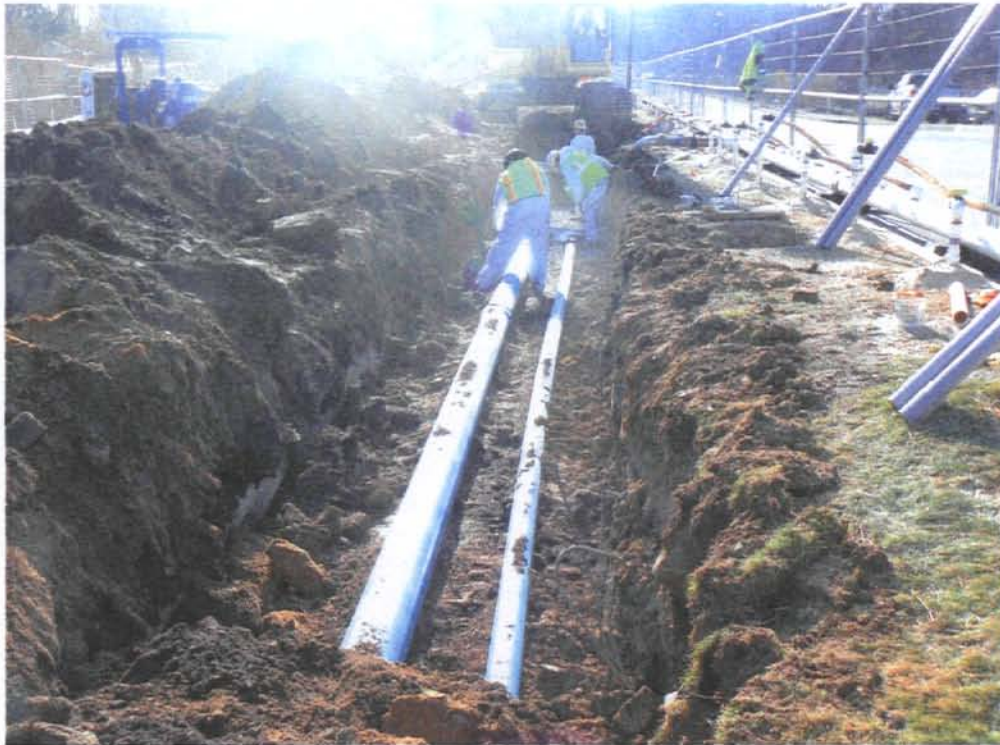
Description: Trench excavation Name: 11Dec2010 004
