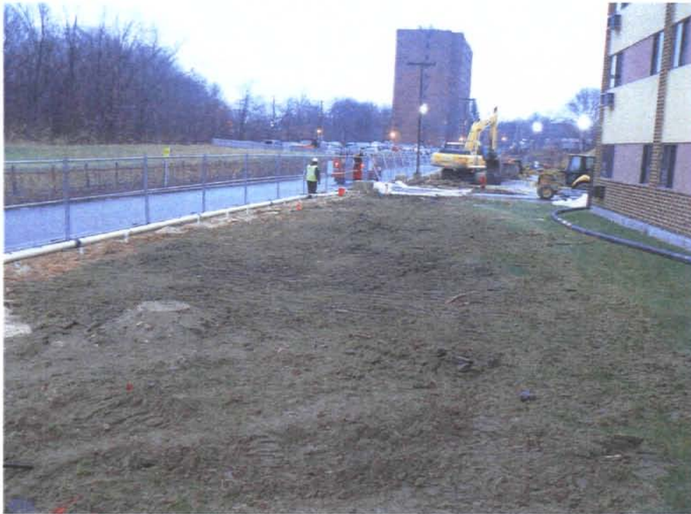
Description: Dewatering components near Centredale Manor building Name: 12Dec2010 001
