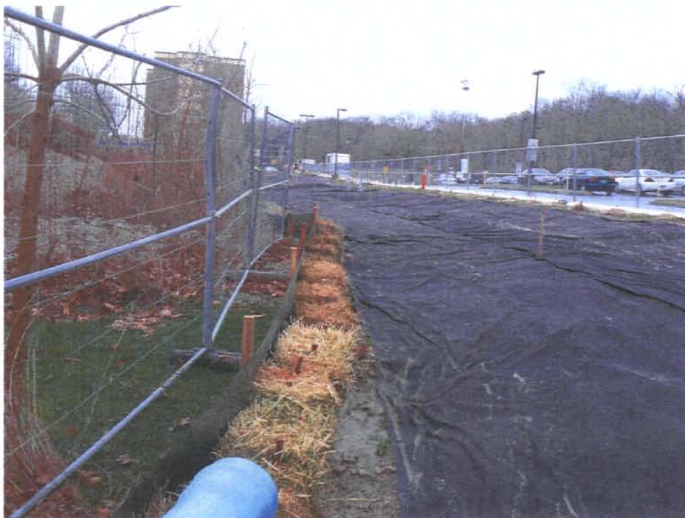
Description: Erosion control haybales Name: 13Dec2010 008
