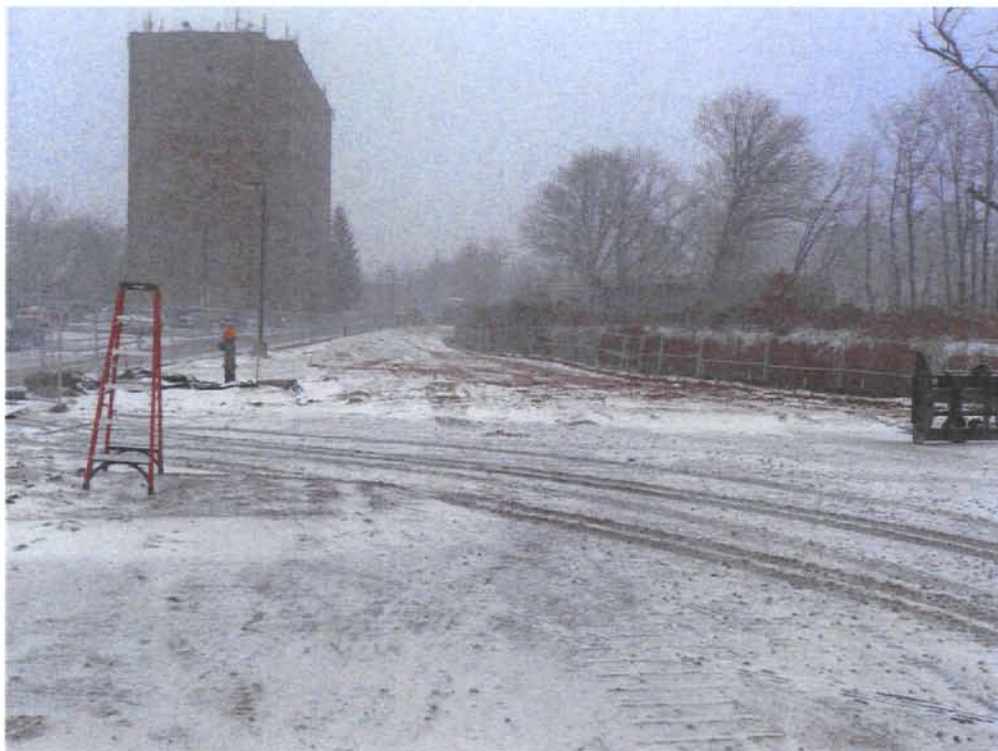
Description: Application of clean fill over trench Name: 21Dec2010 005
