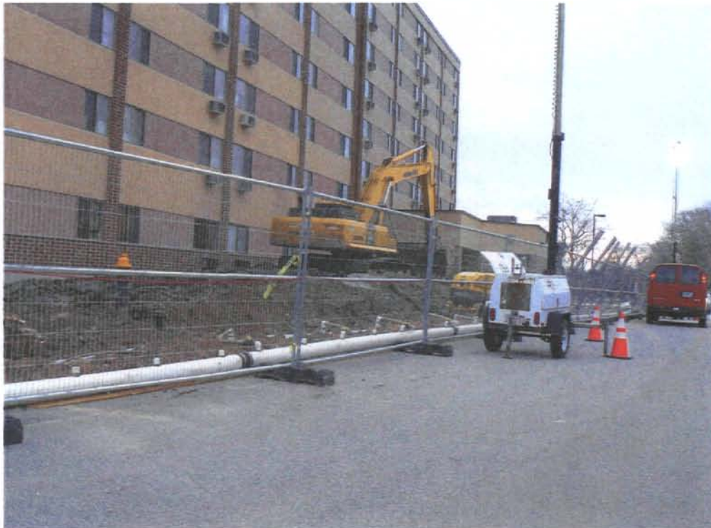
Description: Trenching near Manor building Name: 14Dec2010 001
