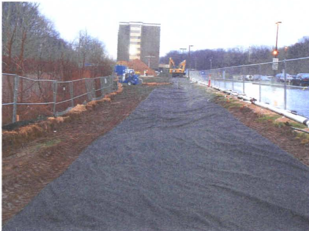
Description: Fabric over completed trench Name: 12Dec2010 019
