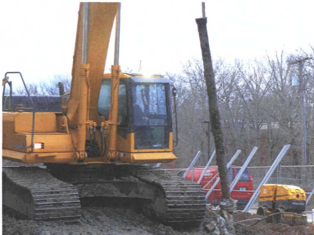
Description: Removal of damaged waterline Name: 14Dec2010 013
