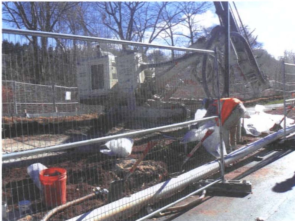
Description: Installation of dewatering components Name: 6Dec2010 019
