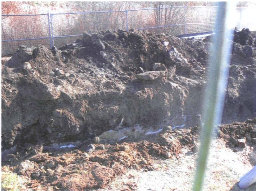
Description: Trench excavation Name: 11Dec2010 002
