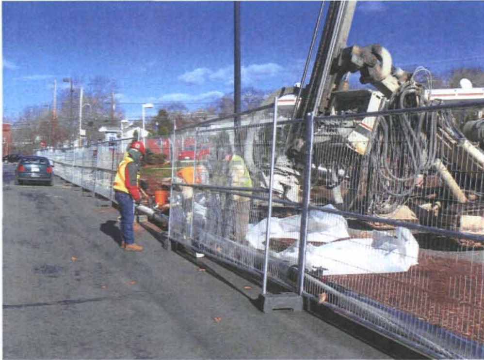
Description: Installation of dewatering components Name: 6Dec2010 021
