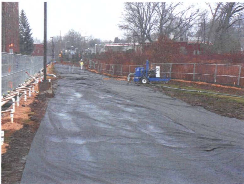
Description: Fabric over completed trench before rain Name: 12Dec2010 033
