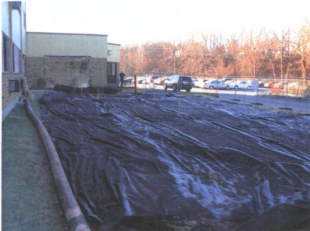
Description: Laying of fabric Name: 17Dec2010 003
