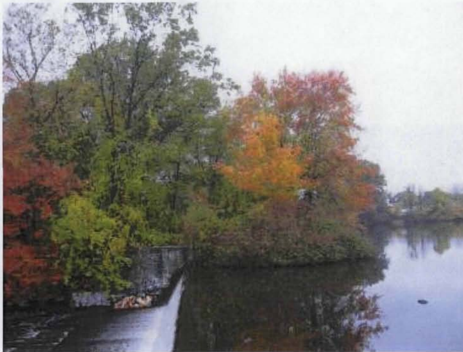
Photo 1: Lyman Mill Pond Dam, viewed from the east, facing west.
