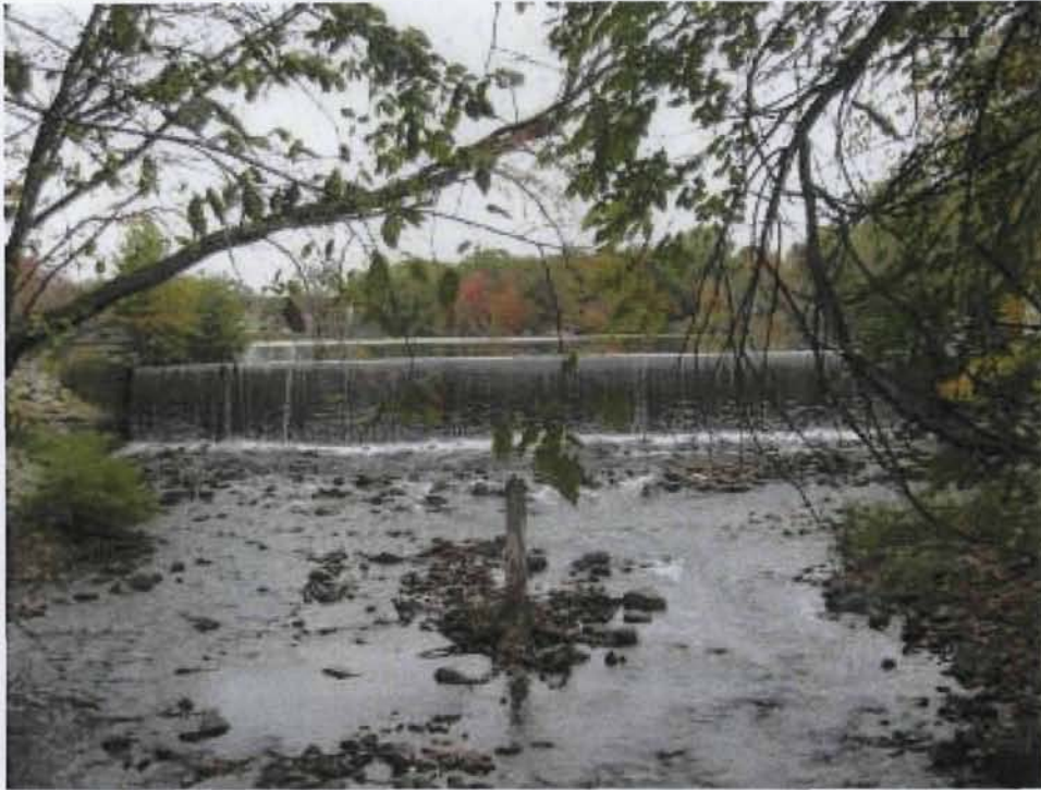
Photo 1: Allendale Pond Dam, viewed from the south, facing north.
