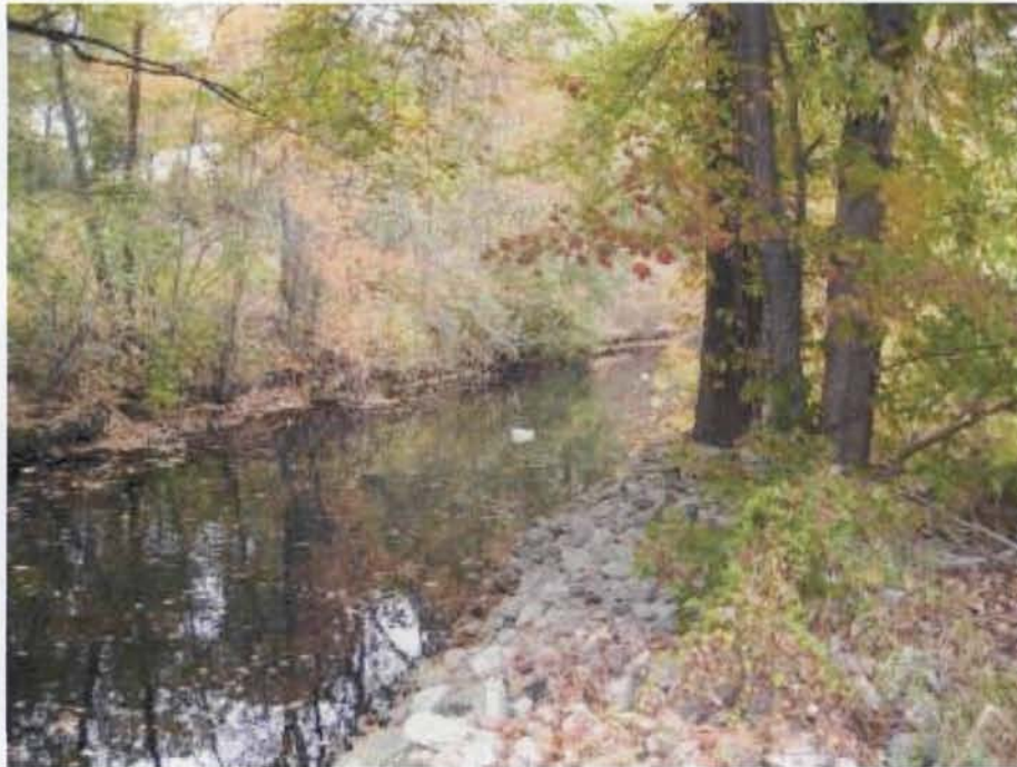
Photo 5: Alternate view of the rip-rap lined portion of the Woonasquatucket River upstream of Allendale Pond, viewed from the east, facing northwest.
