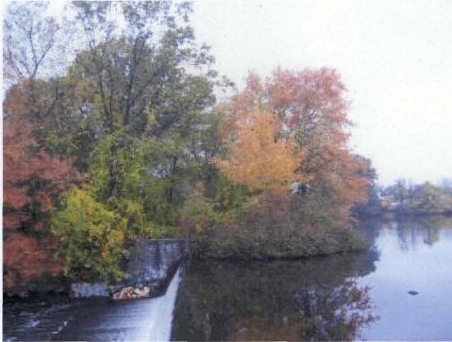
Photo 1: Lyman Mill Pond Dam, viewed from the east, facing west.
