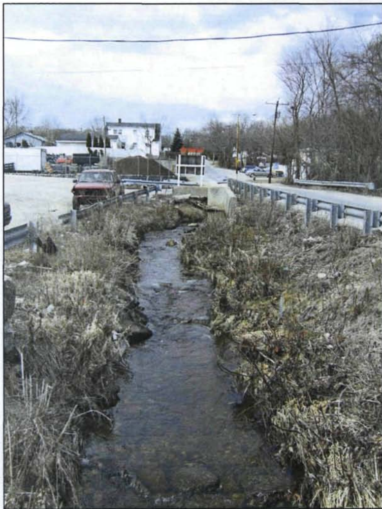
Photograph 16: Assapumpset Brook (looking upstream towards culvert outlet).
