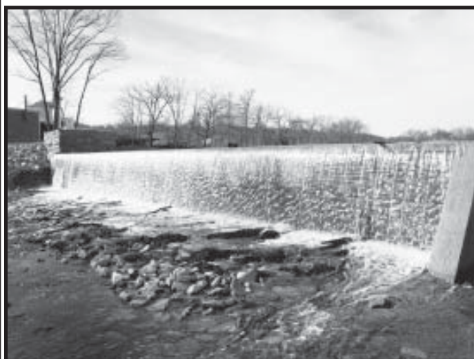
Looking upstream towards the restored Allendale Dam.
