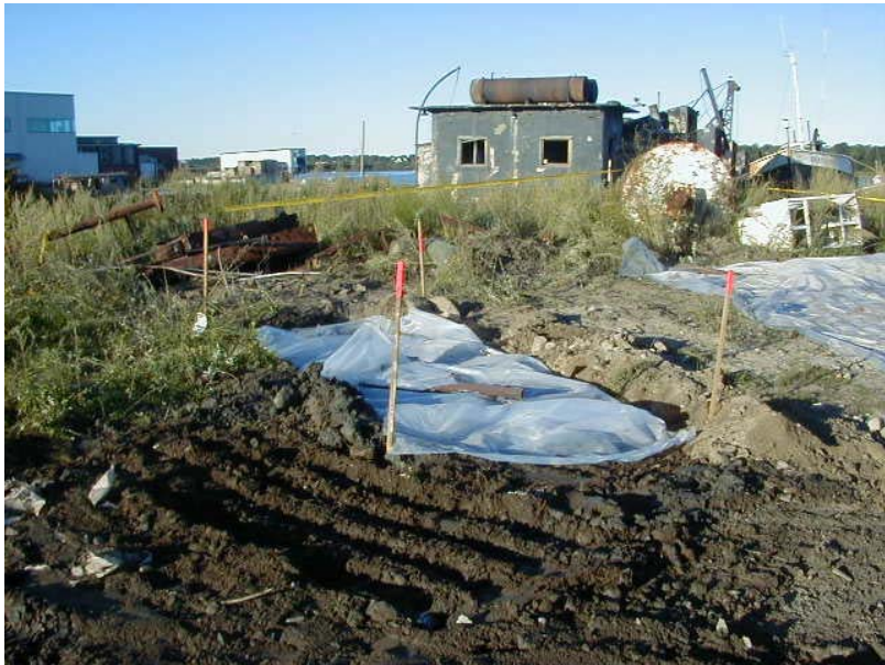
Photo No. 2F: Completed Test Pit (TP-D3)
