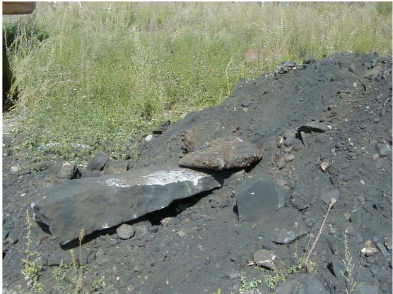
Photo No. 5A: Steel and Concrete Debris (TP-D16)
