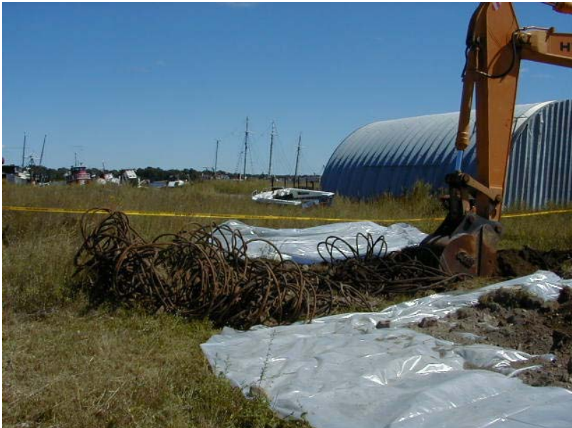
Photo No. 2B: Steel Cable Coil (TP-D2A)
