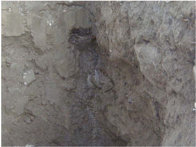
Photo No. 3D: Groundwater Seep
