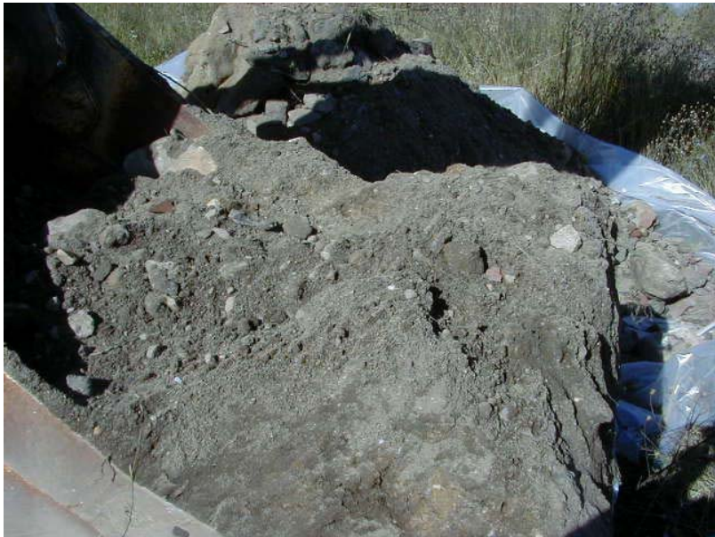
Photo No. 1C: Excavated Material (4-4.5')
