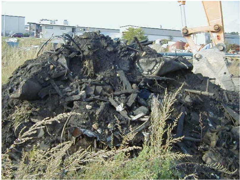
Photo No. 6D: Excavated Debris
