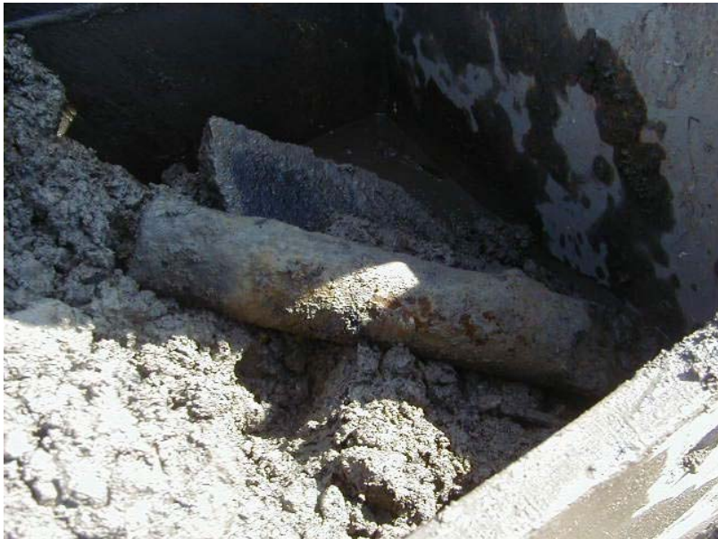
Photo No. 5C: Piece of Steel Debris (TP-D17)
