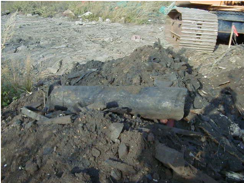
Photo No. 6B: Section of Steel Pipe Filled With Concrete
