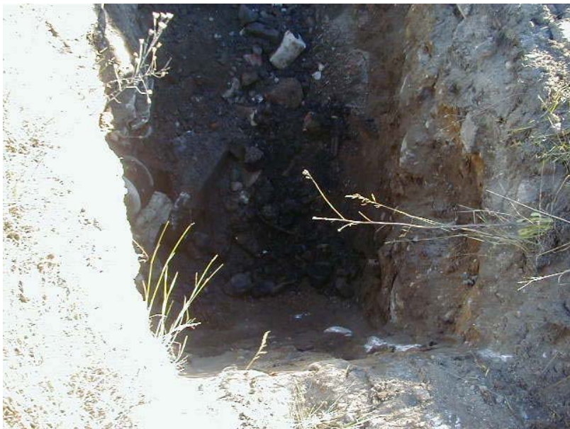
Photo No. 1F: Completed Test Pit
