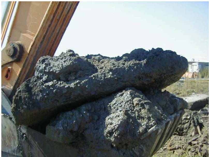
Photo No. 4D: Asphalt and Concrete Debris Layer (TP-D14)
