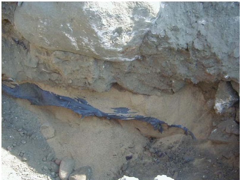
Photo No. 7D: Layer of Polyethylene Plastic and Sand (TP-D10)
