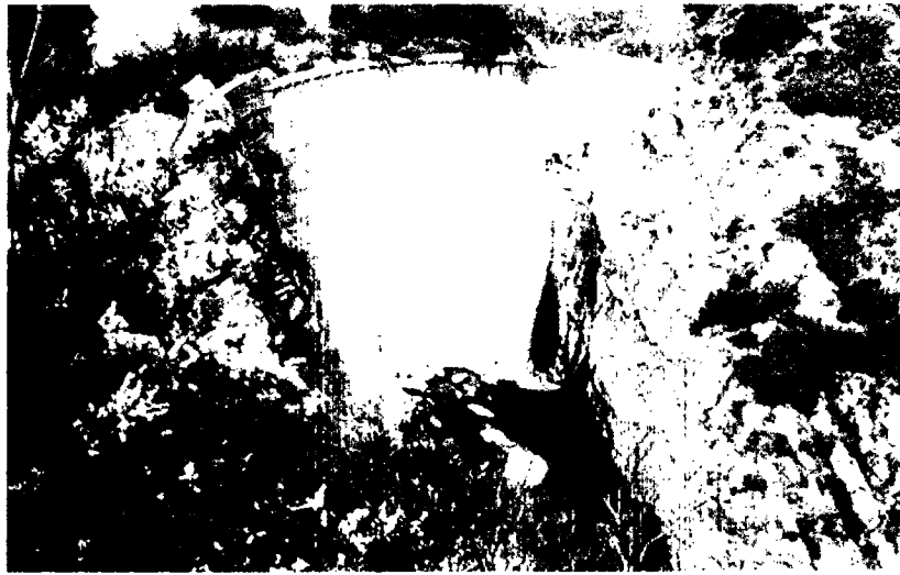
Figure 1.6 Rindge Dam, built in the 1920s on Malibu Creek in California, is an example of a concrete arch dam. Courtesy of Sarah Bairn.
