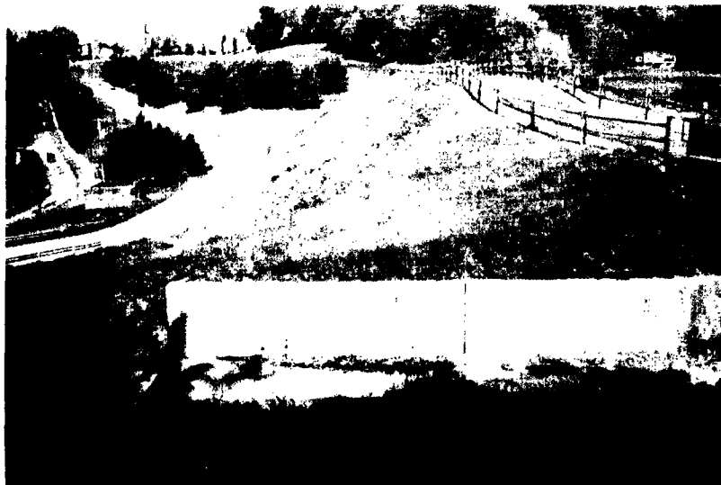
Figure 1.4 Township Line Dam, across Township Line Run in Pennsylvania, is an example of an earth fill dam. Courtesy of the Pennsylvania Department of Environmental Protection.
