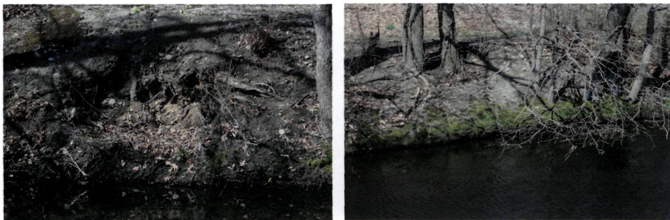
Figure 3. View looking toward the western bank of the Woonasquatucket River, adjacent to the source area, April 18, 2006. Left – the disturbed area in the central portion of the photograph appears to be where a tree had been up-rooted. Right – evidence of abundant, thick moss growth.
