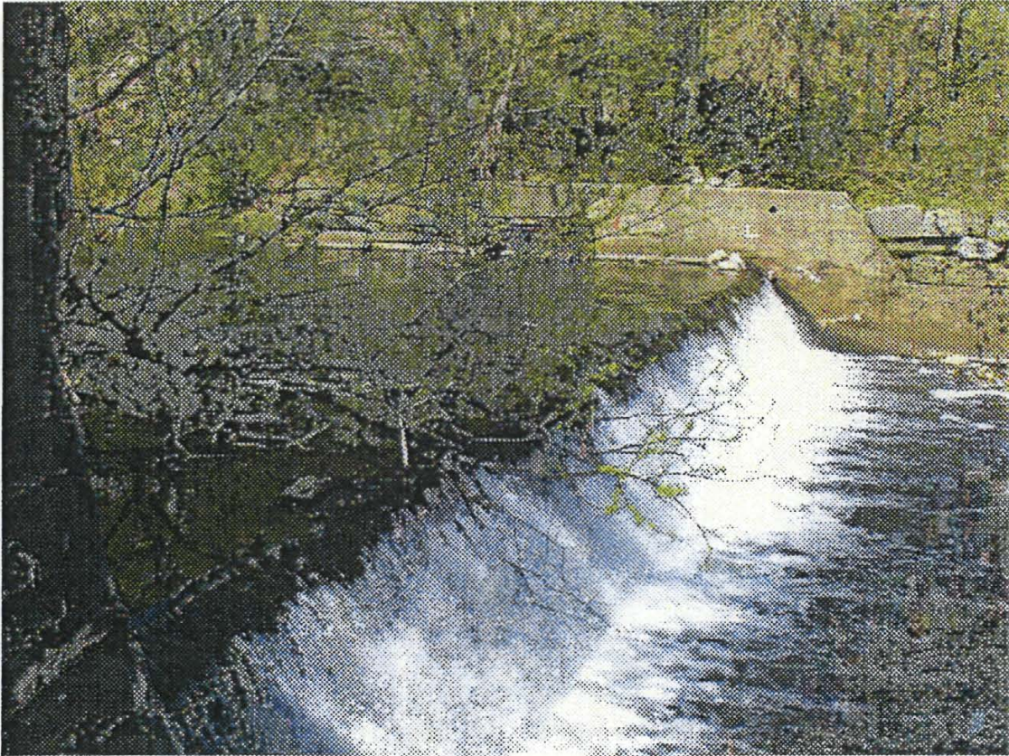
Photo 1 – Overview of dam from right bank.
