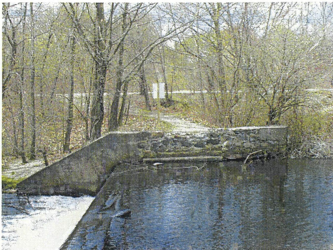
Photo 1 – Overview of right embankment from left.
