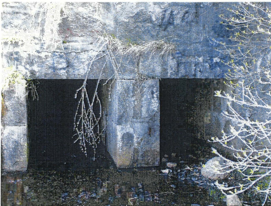
Photo 6 – Downstream end of outlet works on left side of spillway.
