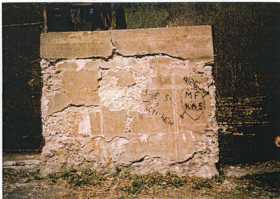
Photo 1: Extensive spalling and concrete deterioration of the gate operator stand at the right side of the spillway.
