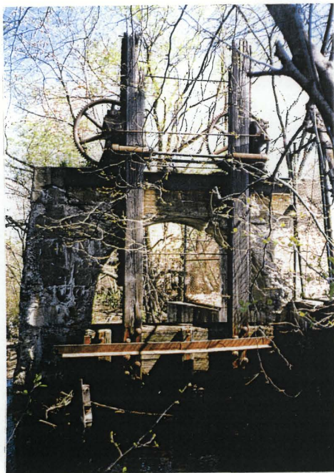
Photo 1: Extensive spalling and concrete deterioration of the gate operator stand at the right side of the spillway.
