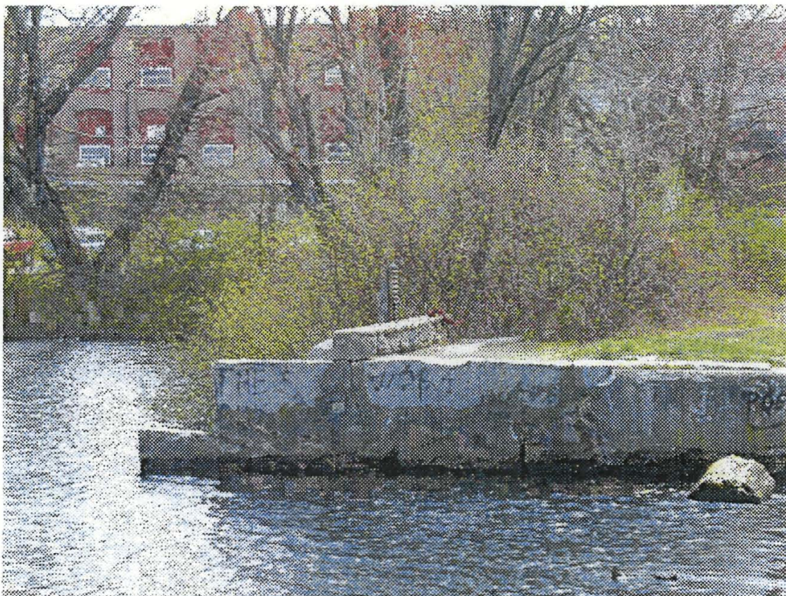
Photo 5 – View of outlet works on left end of spillway.
