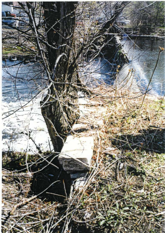
Photo 5: Missing 2x8 timber at the left side of the spillway, allowing water to flow over the spillway.
