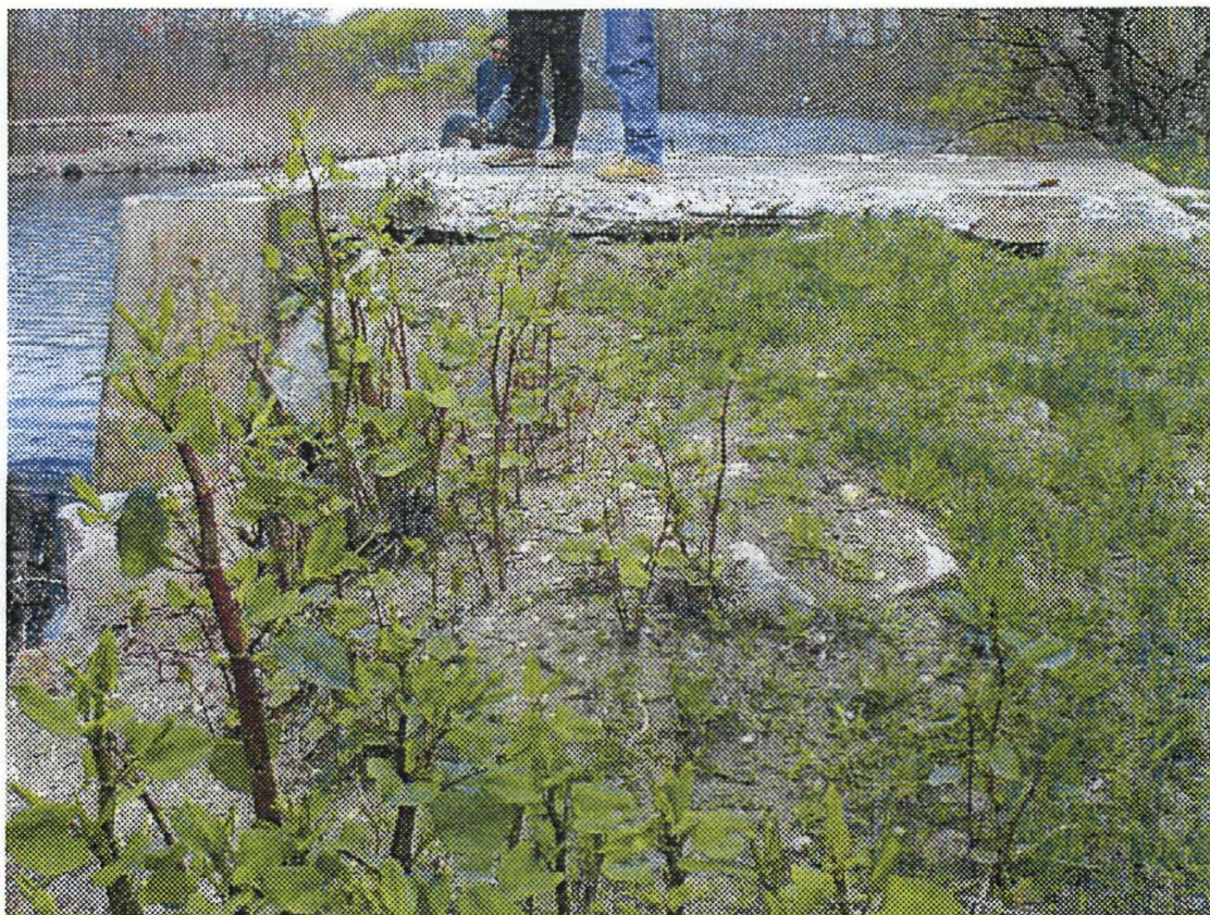
Photo 5 – Soil filling downstream side of outlet works.
