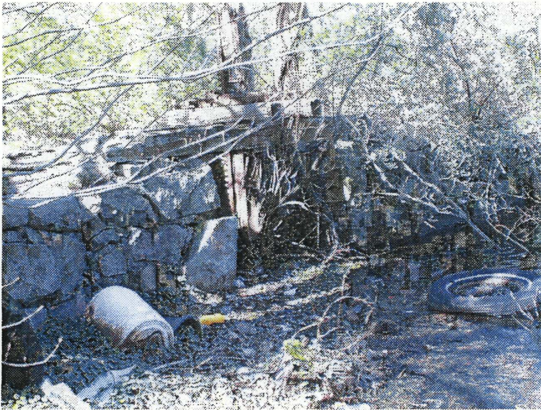
Photo 4 – Outlet works on left bank.
