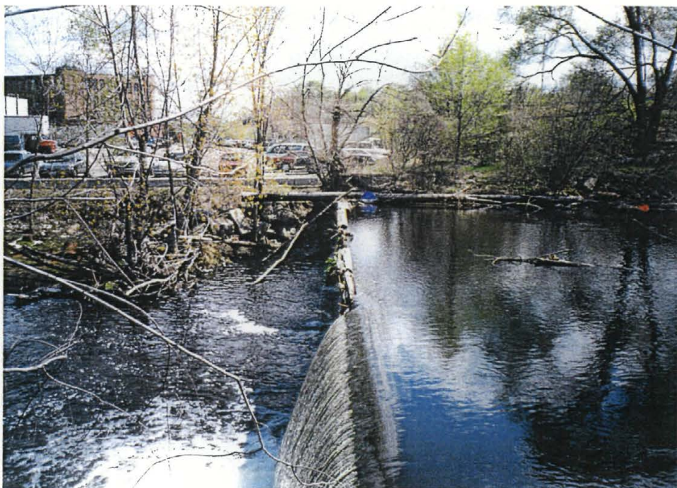
Photo 5: Missing 2x8 timber at the left side of the spillway, allowing water to flow over the spillway.
