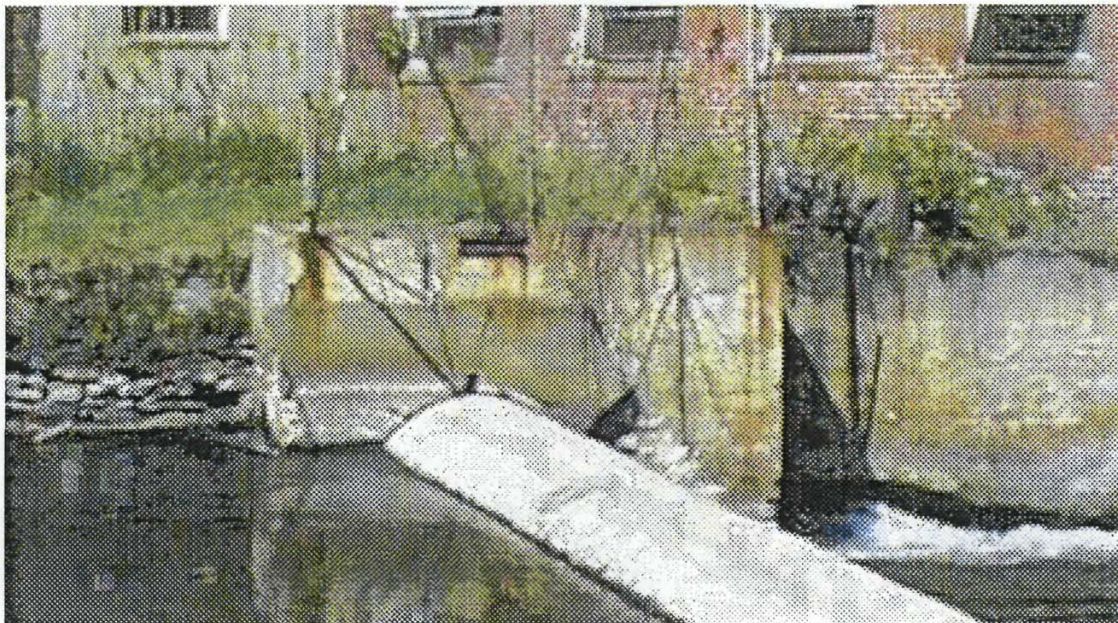
Photo 5 – Outlet works on left side of spillway.
