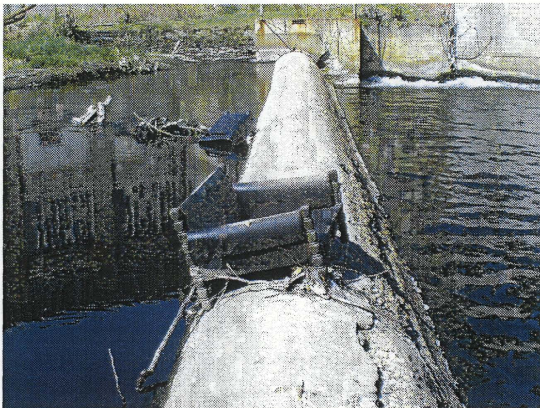
Photo 3 – Spillway from right bank.
