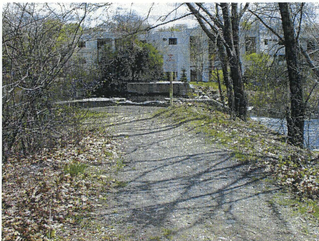
Photo 2 – Overview of right embankment looking towards spillway.
