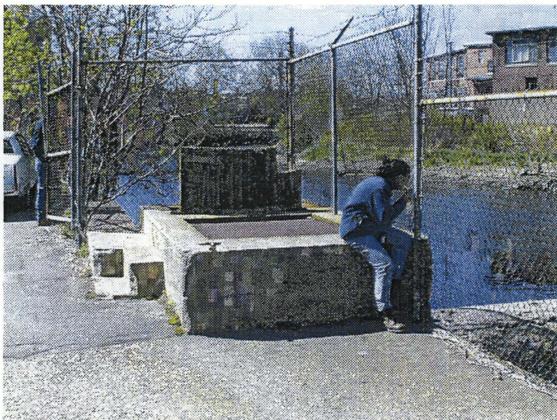
Photo 4 – Outlet works on right bank with raised wooded gate.
