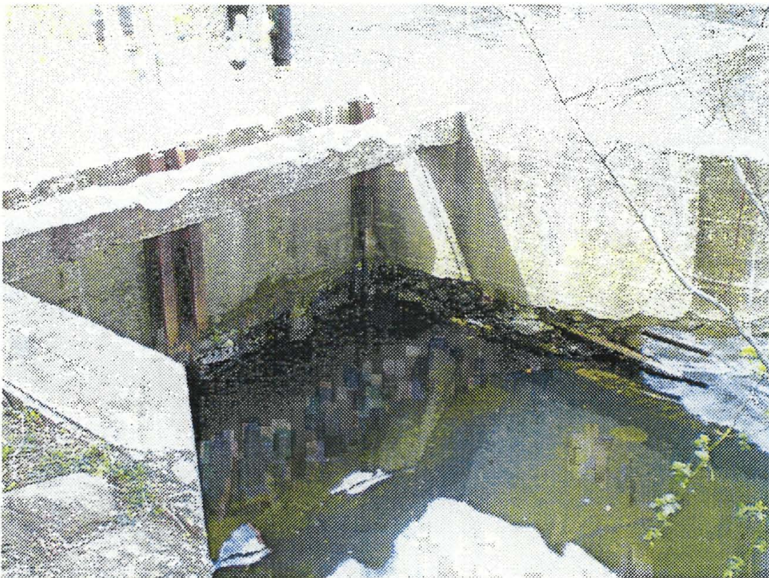
Photo 4 – Inlet to outlet works at left end of spillway.
