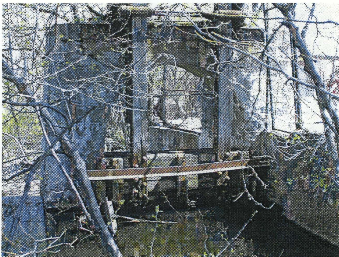
Photo 4 – Upstream view of outlet works on right bank.
