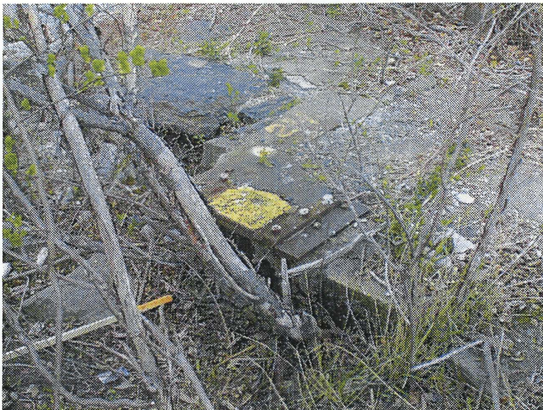
Photo 3 – Outlet works are filled in with earth.
