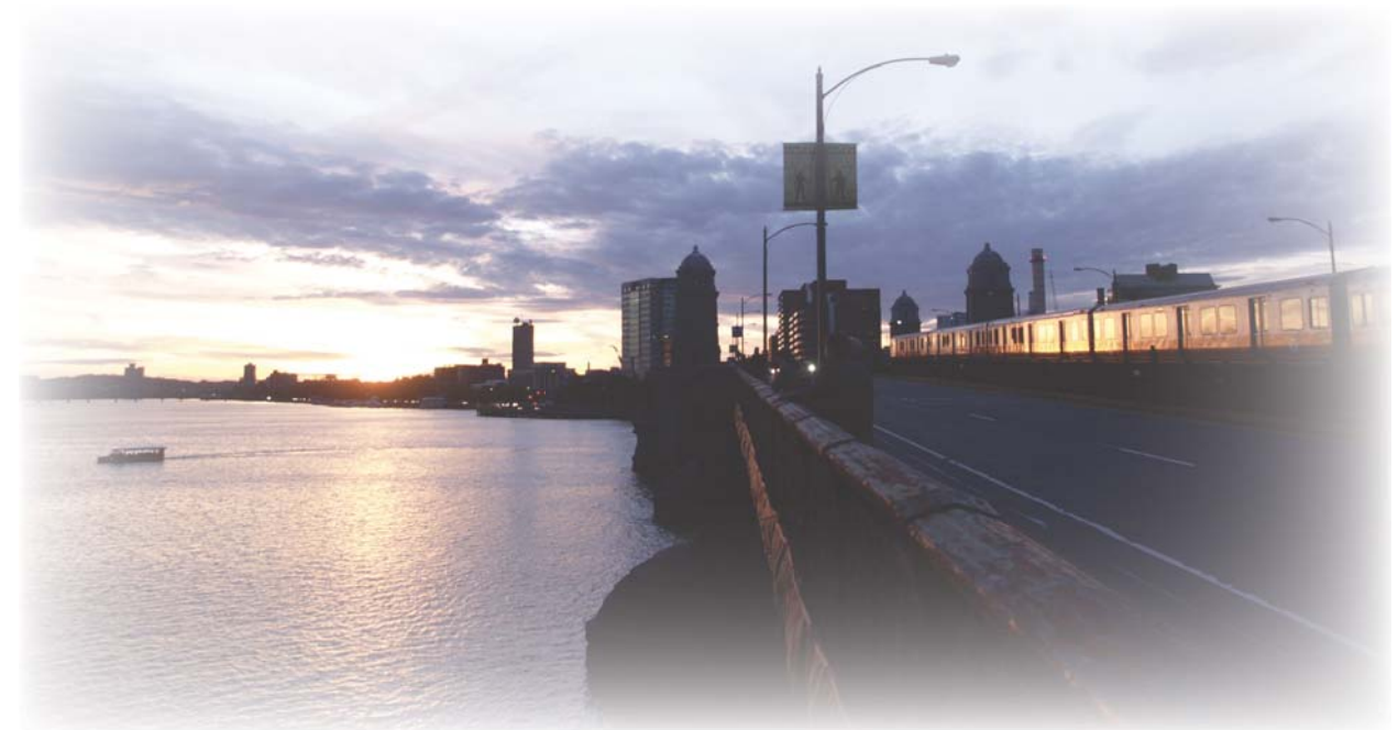
Longfellow Bridge over the Charles River, Boston MA (photo: Roy Crystal)
