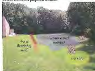
Figure 2. Gravel based wetland system with underground chambers, pretreatment sediment forebay, and retaining wall.
