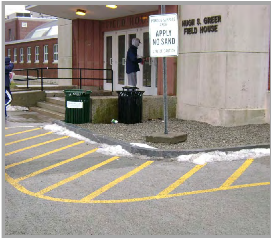
Field House Pervious Concrete Lot
