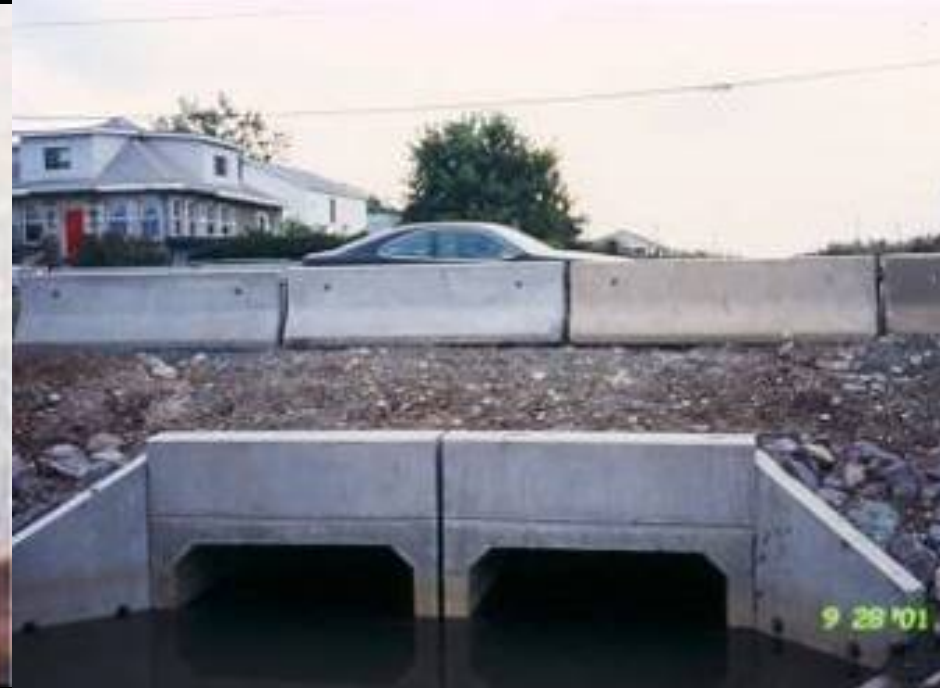
New Twin Box Culvert (adequate flow)
