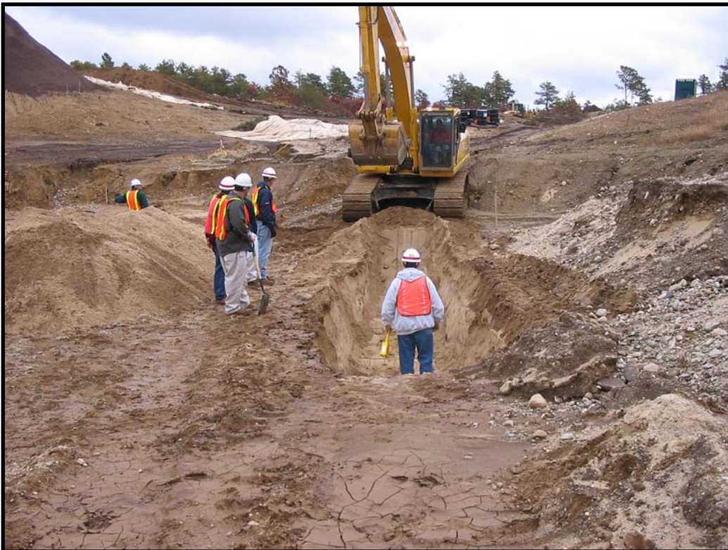
Photograph 3-8 Excavation of test trench
