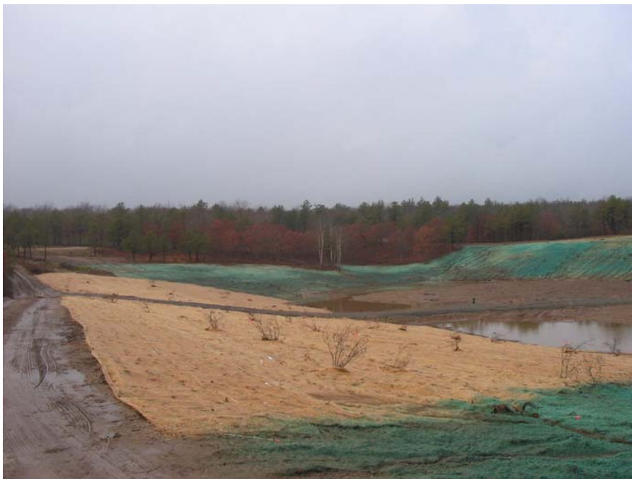
Photograph 4-2 Demo Area 1 – Graded and backfilled
