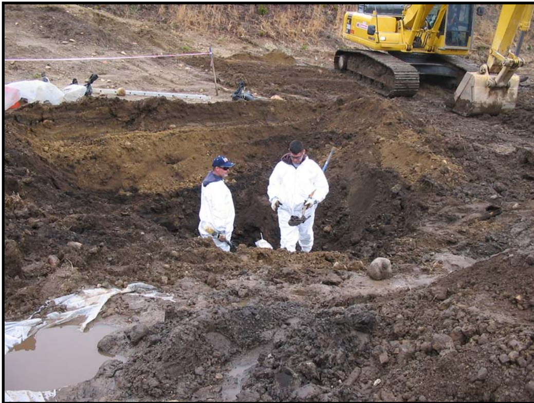
Photograph 3-10 Items being removed from burn pit
