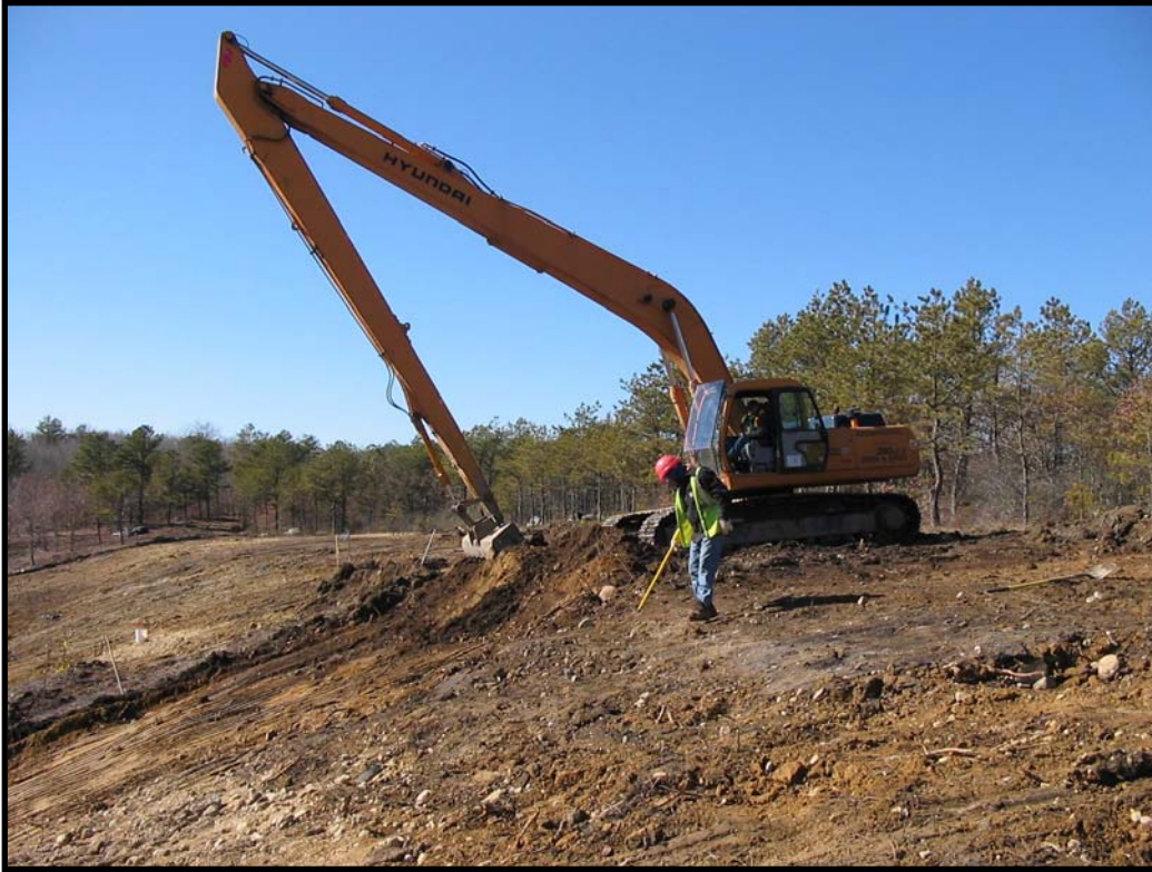
Photograph 3-7 UXO personnel were present during all excavation activities
