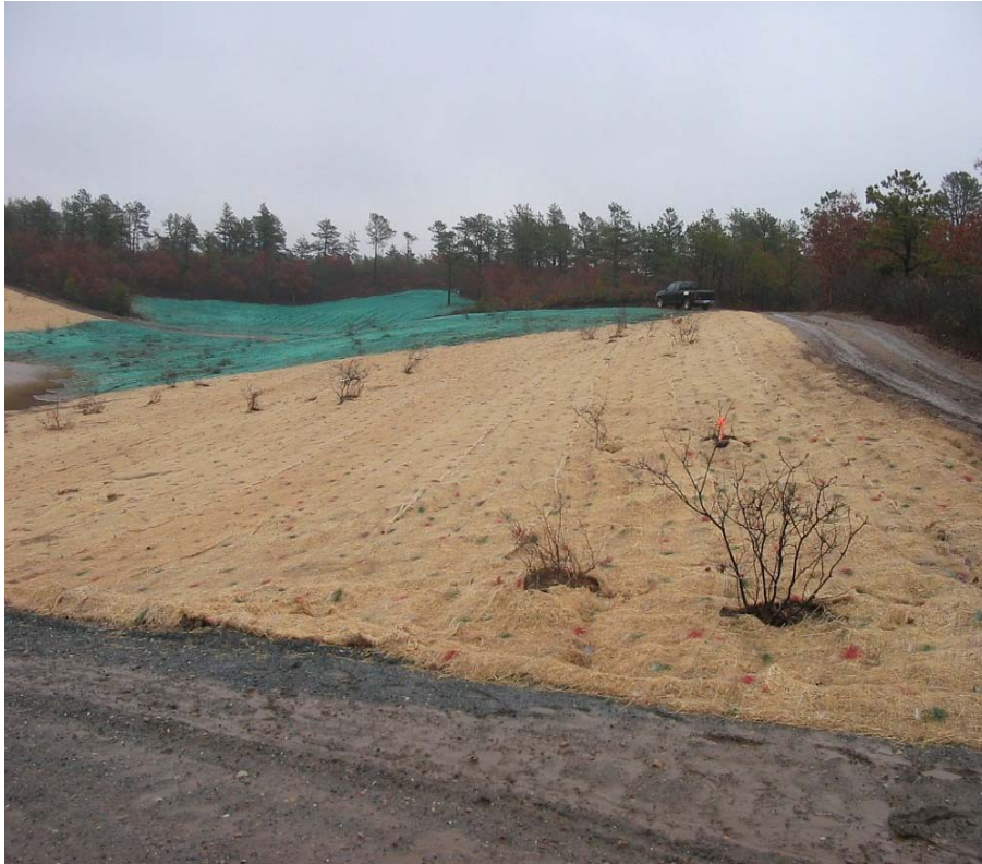
Photograph 4-1 Demo Area 1 – Erosion control and vegetation
