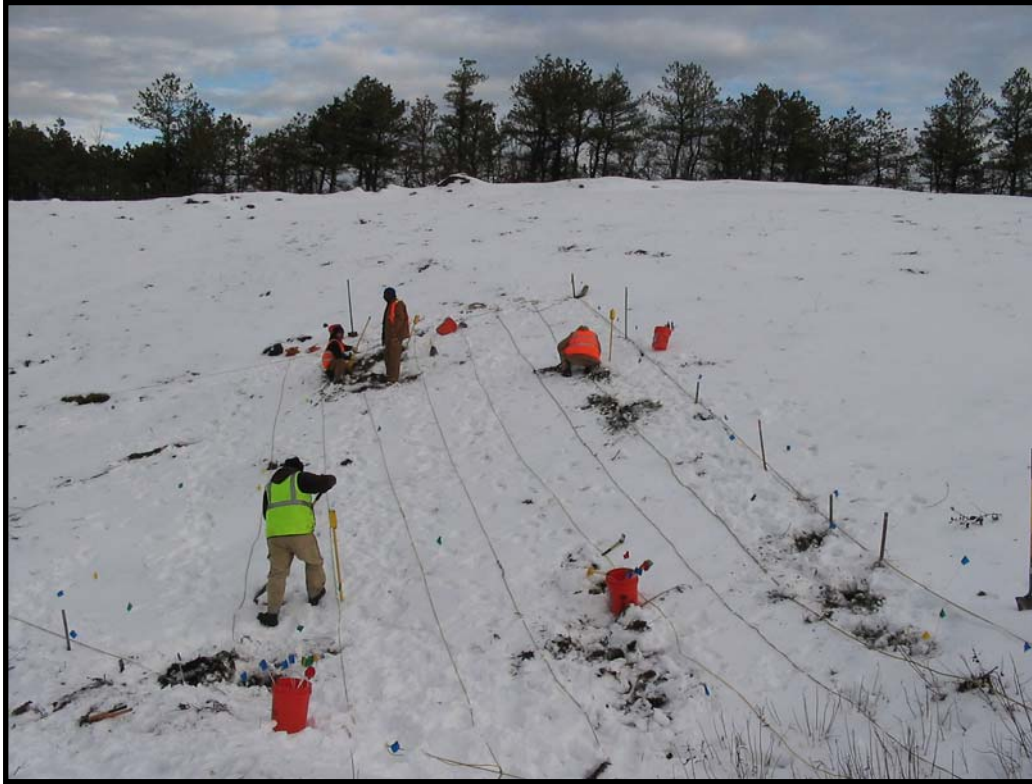
Photograph 3-1 Pre-excitation UXO clearance by grid
