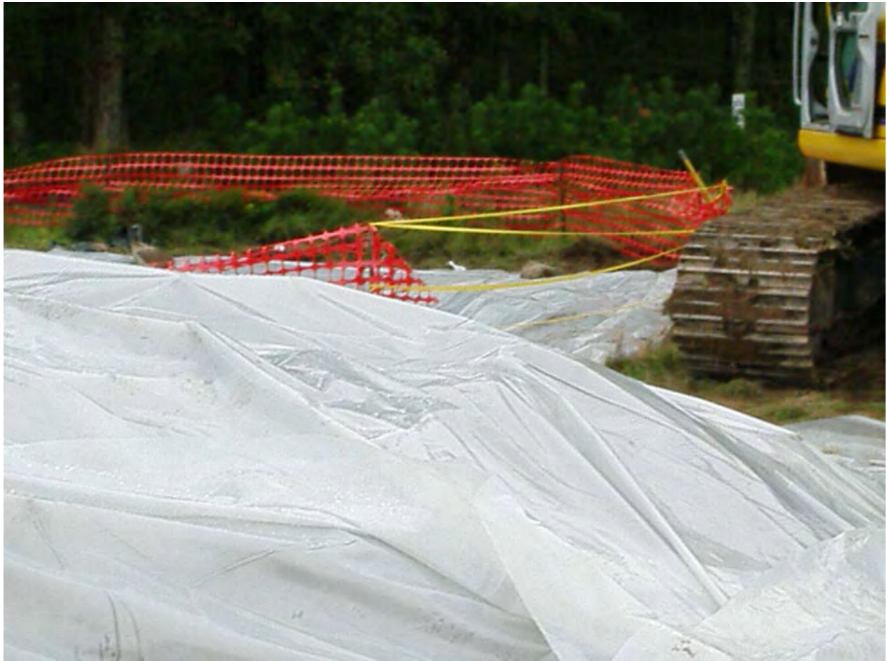
Photo 4: Construction Fence Around Excavation Area
