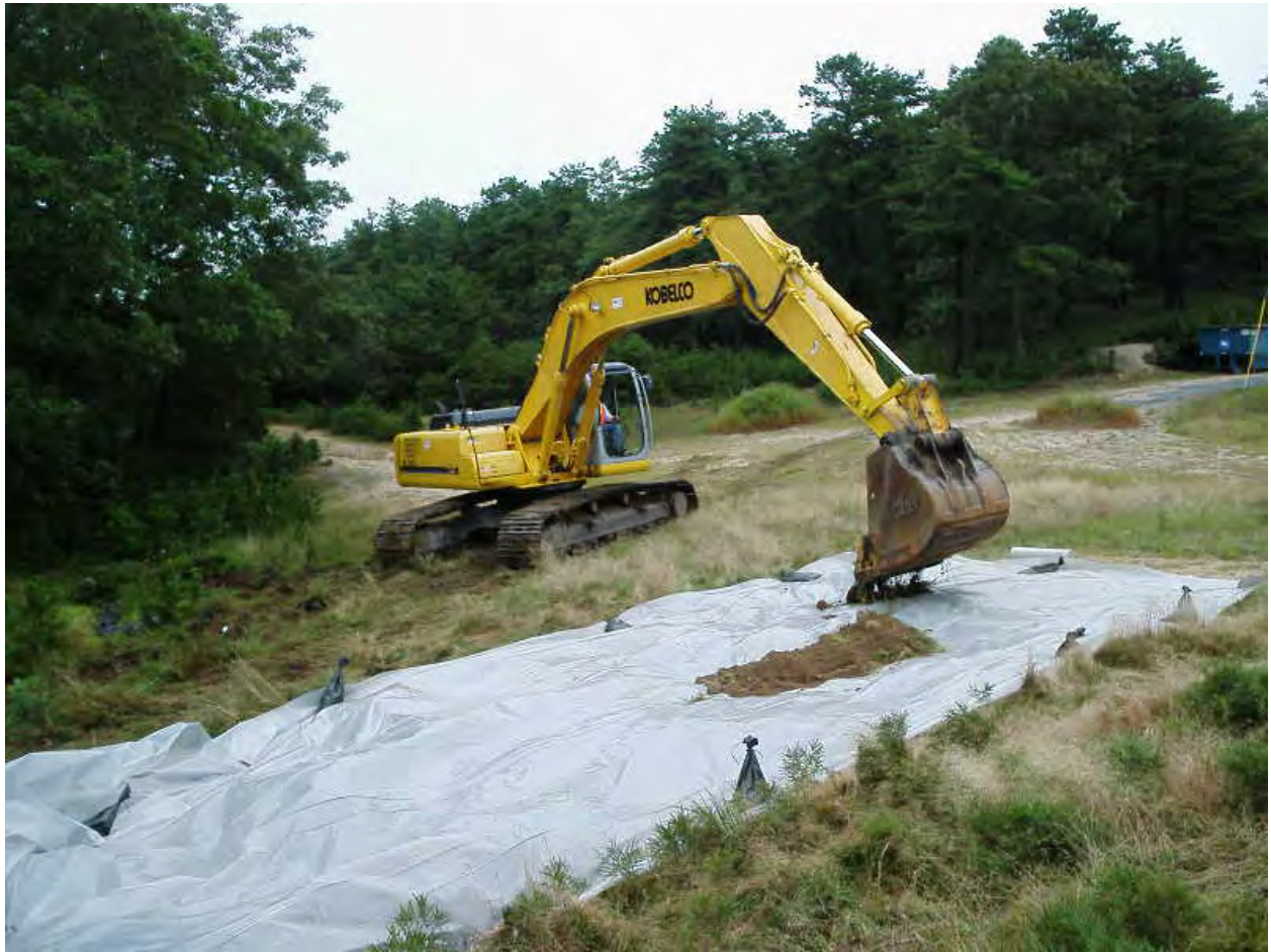
Photo 2: Soil Stockpile Area
