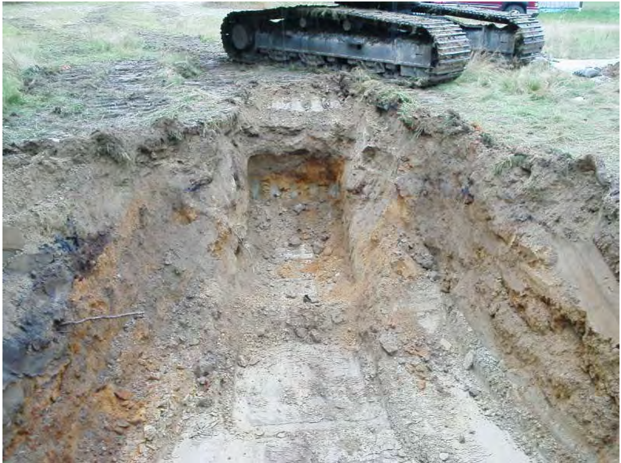
Photo 1: Area A Excavation
