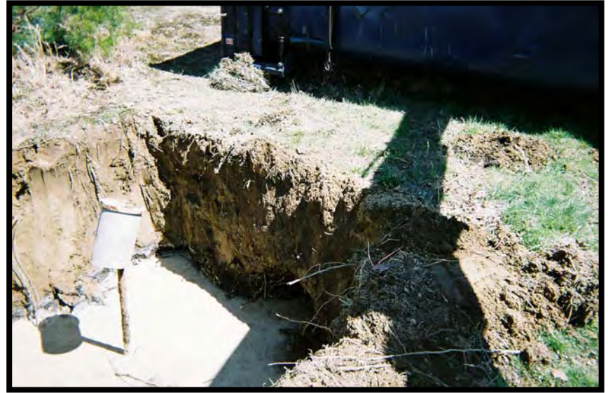
Photo 7: Area E Excavation
