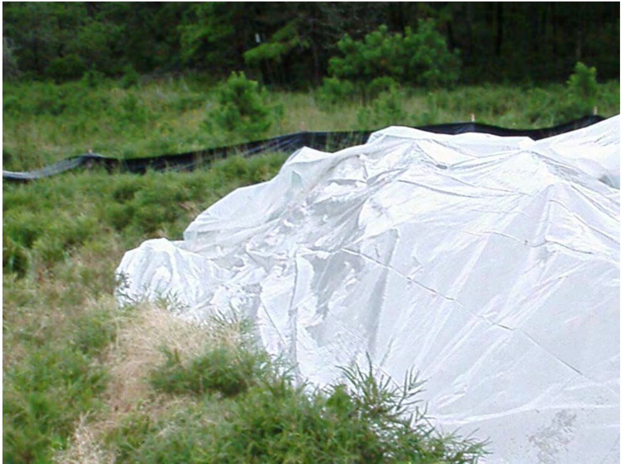
Photo 3: Covered Soil Stockpile and Silt Fence
