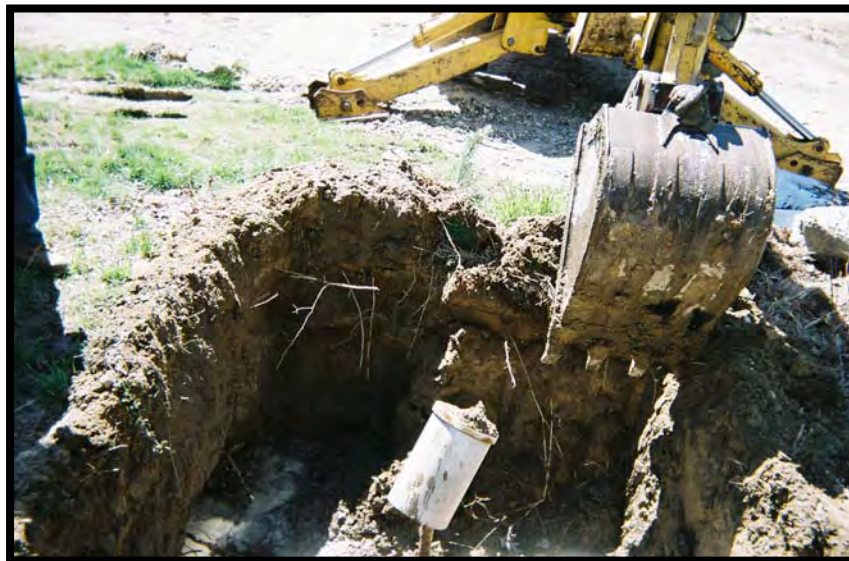
Photo 12: Area E Excavation
