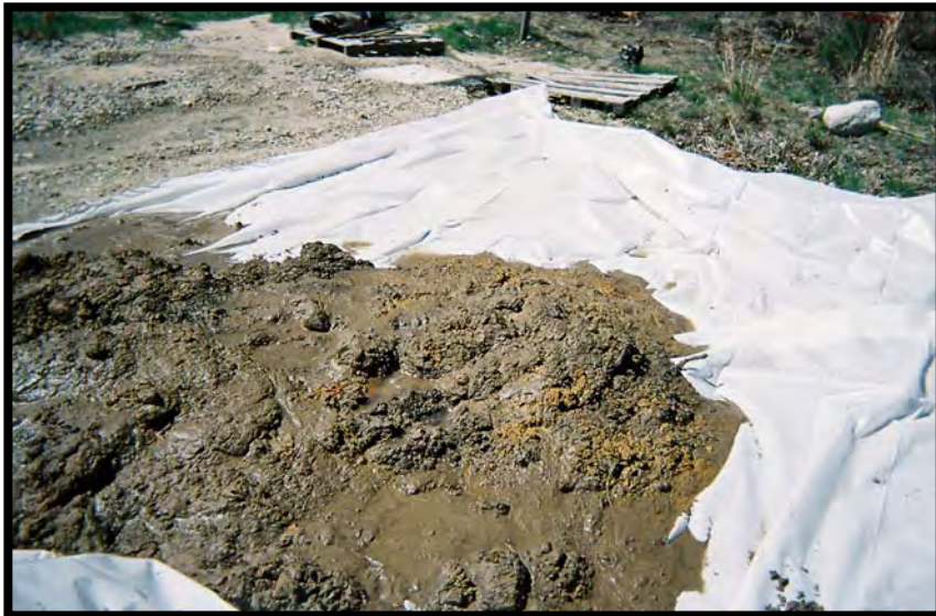
Photo 10: Soil Stockpile Area
