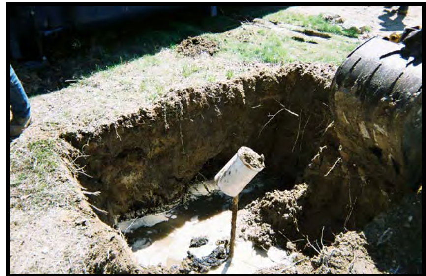
Photo 13: Area E Excavation
