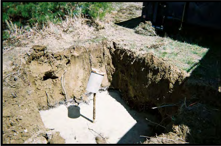
Photo 6: Area E Excavation
