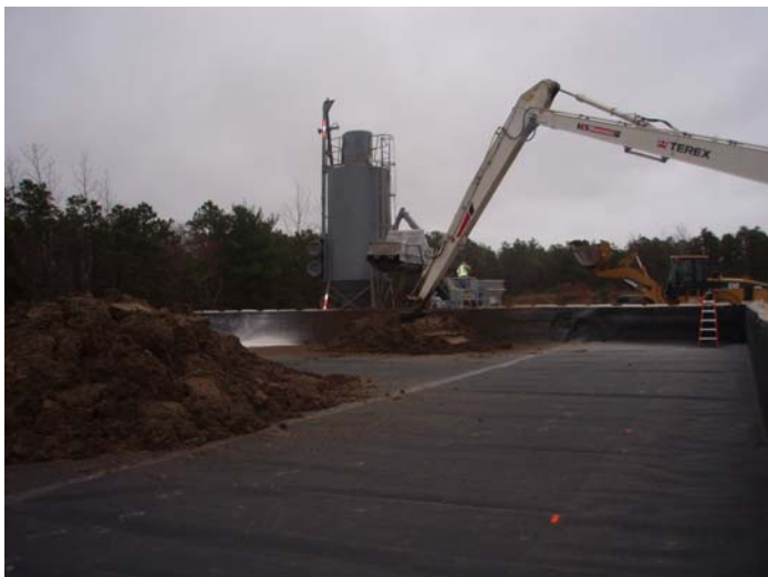
Soil treatment operations – winter 2009
