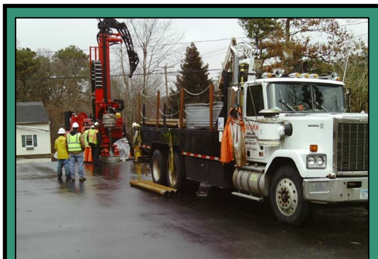
A sonic drill rig and tender vehicle
