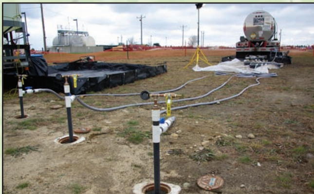
In situ chemical oxidation operation
