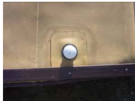
Figure 4-6. Port Access for Water Inspection and Removal
