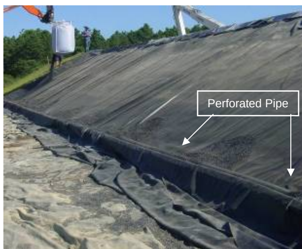
Figure 3-4a Liner with Perforated Pipe
