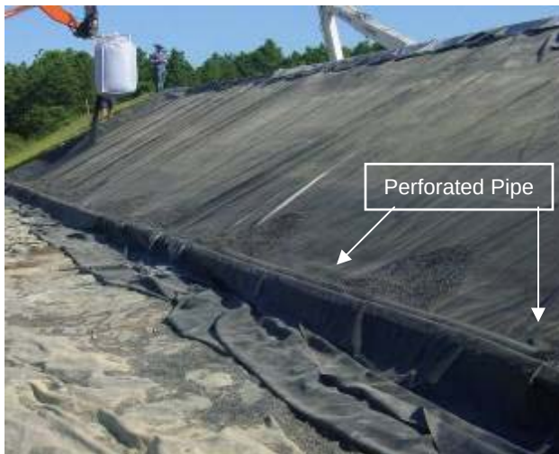
Figure 3-3a. Liner with Perforated Pipe
