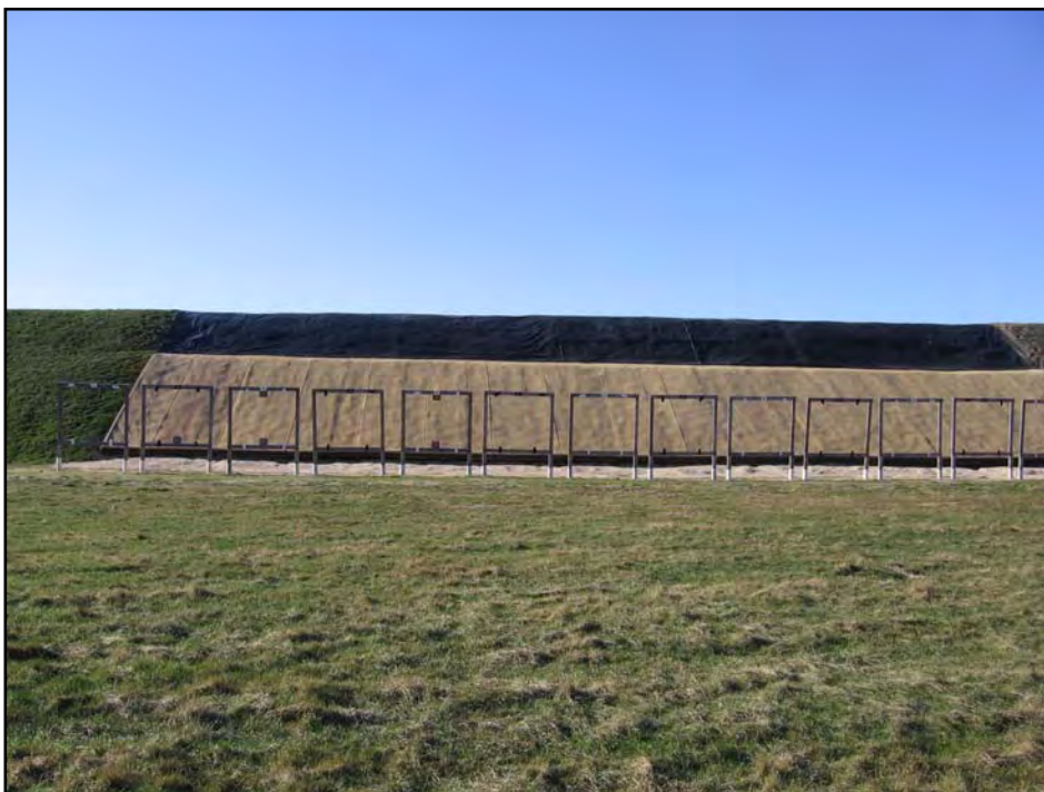
Photo 06: Facing south at the central portion of berm.
