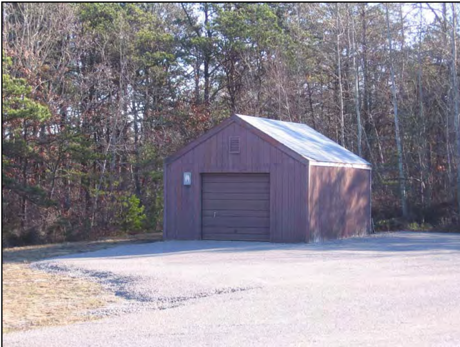
Photo 04: The storage shed located at the northeastern corner of the gravel drive.
