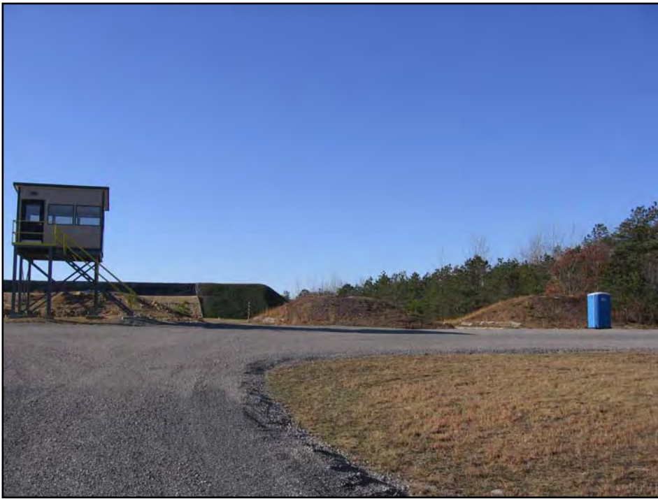
Photo 03: Facing southwest at the firing range from the northern access road.
