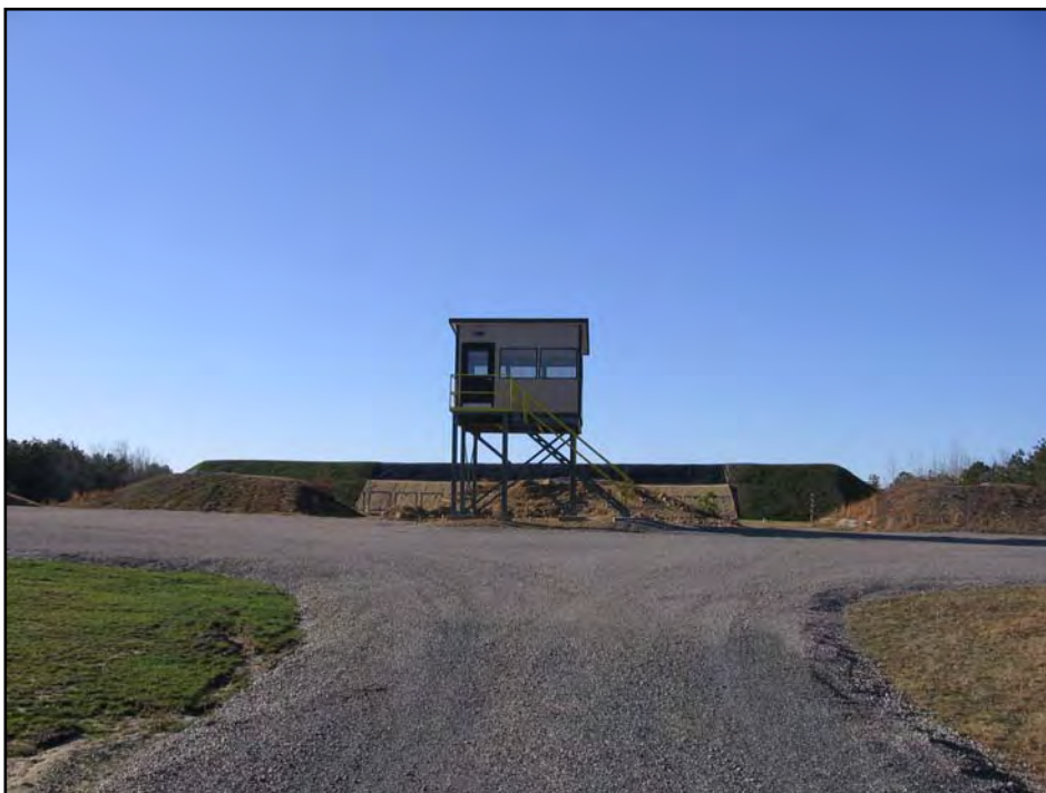
Photo 02: Facing south at the firing range from the northern access road. Note the tower and berm built August/September 2006.
