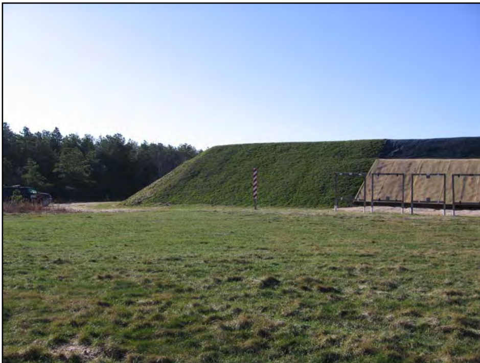
Photo 05: Facing southeast at the eastern portion of the berm. Photos 05-07 are a panoramic of the entire berm.
