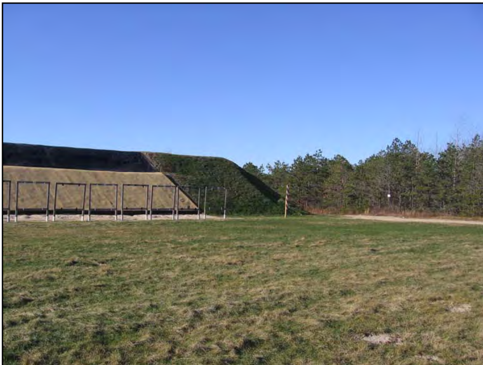
Photo 07: Facing southwest at the western portion of the berm.
