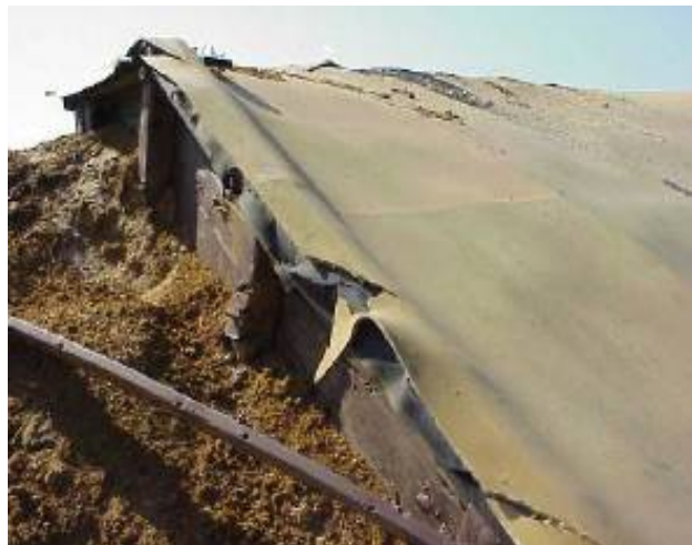
Figure 6-4. Example of Damage to STAPP™ Support Frame
