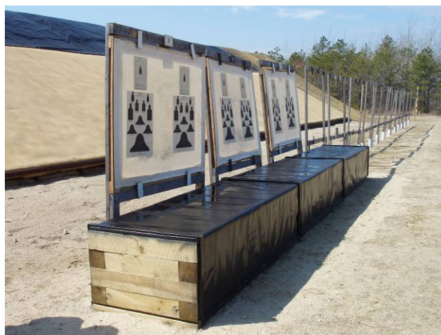
Figure 5-2. Protective Sand Boxes and Target Frames on T Range
