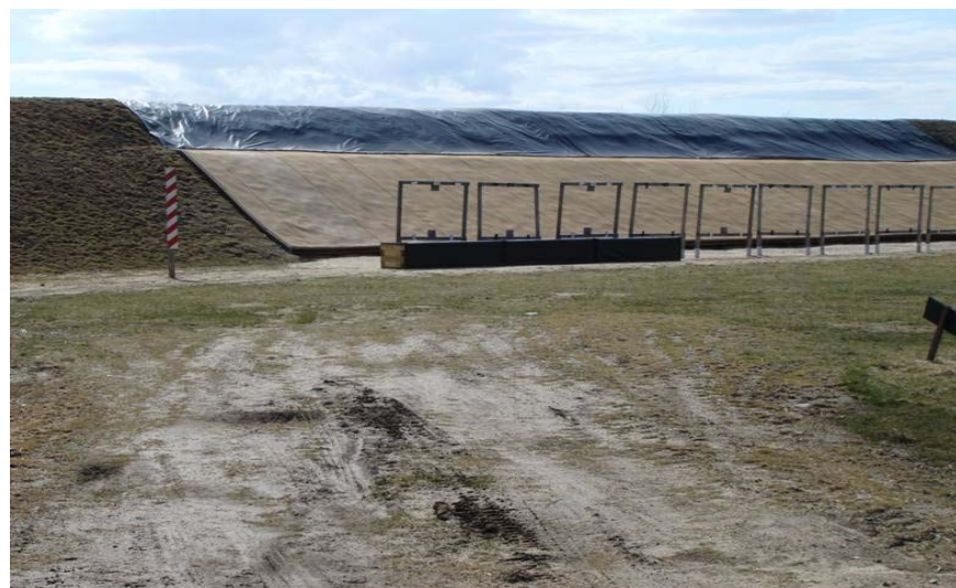
Figure 5-3. STAPP System and Geotextile Tarp on T Range
