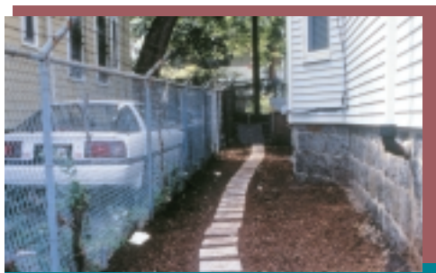
Install stepping stones to prevent contaminated soil from being tracked into the house.
