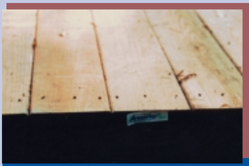
Wood platform built with ACQ lumber.
