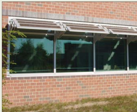
Photovoltaic window shades produce energy
