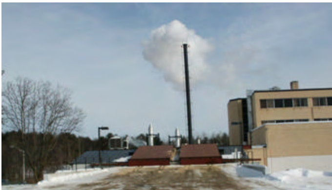
North Country Hospital fuel storage, boiler plant, and tall stack
