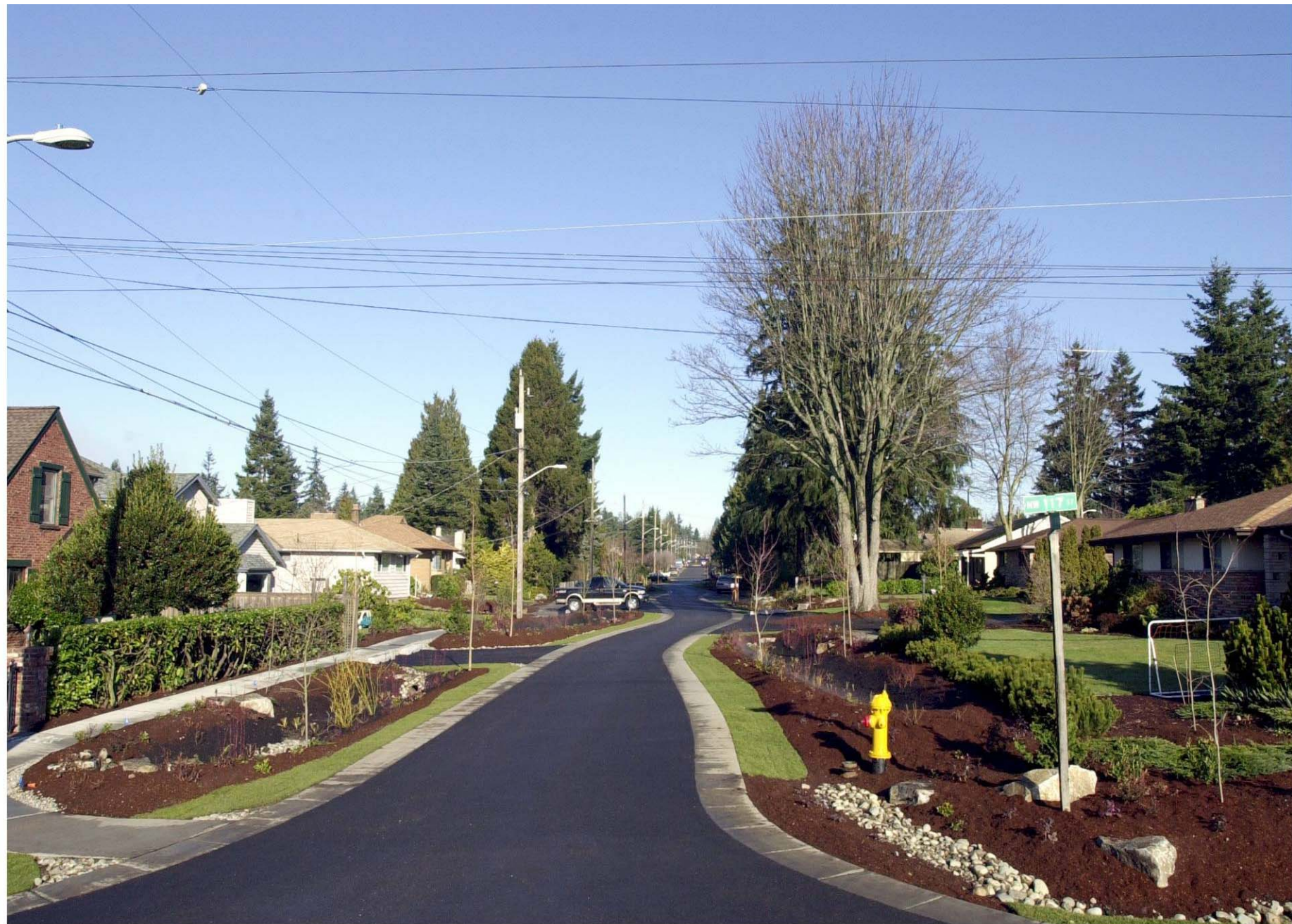
After Completion - January 2001
