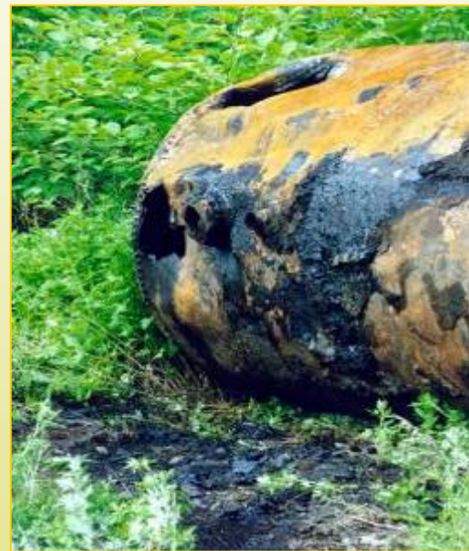
UST removal at Riverside Hills, Providence, RI
