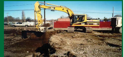
Workers clean up petroleum at a brownfields site in Prineville, Oregon.
