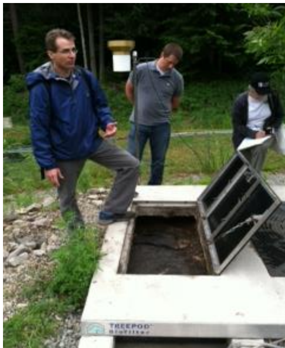
Tree Filter system shown, with James Houle, Principal Investigator, University of New Hampshire, Stormwater Center. Team includes EPA's Office of Research and Development, Edison NJ.
