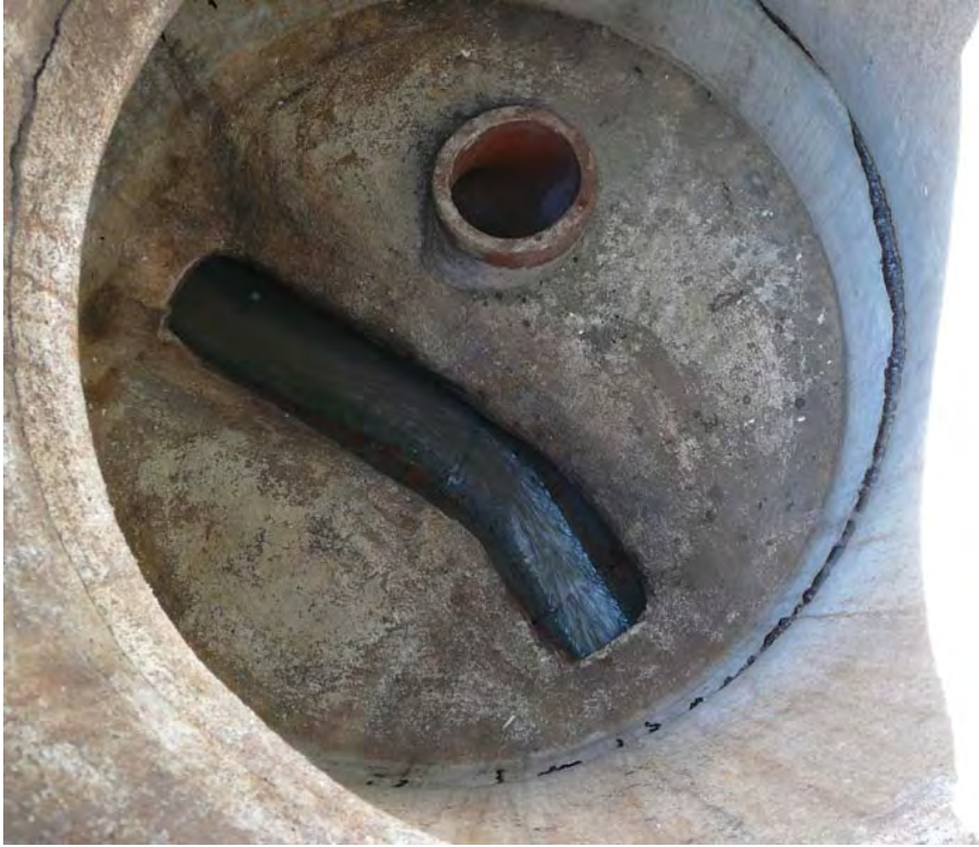
Photo 7 "Stanford & Wellesley" - Addition of underflow pipe to prevent overflows from this manhole
