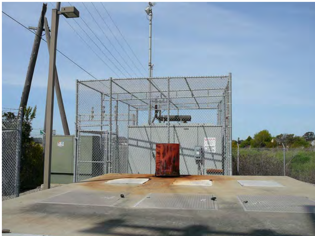
Photo 2 Generator for Burlingame pump station
