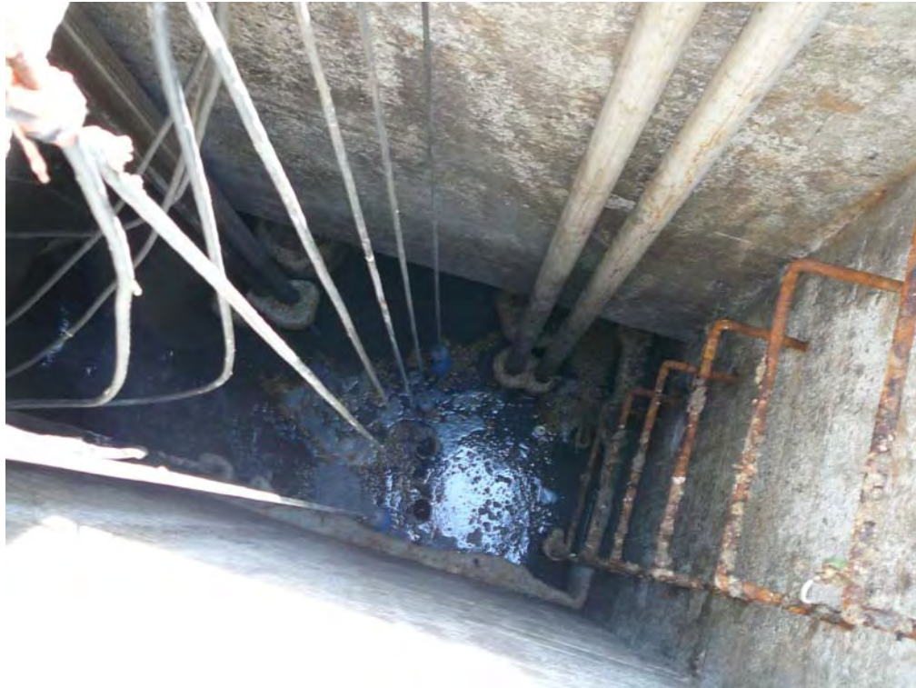
Photo 1 Burlingame pump station wet well
