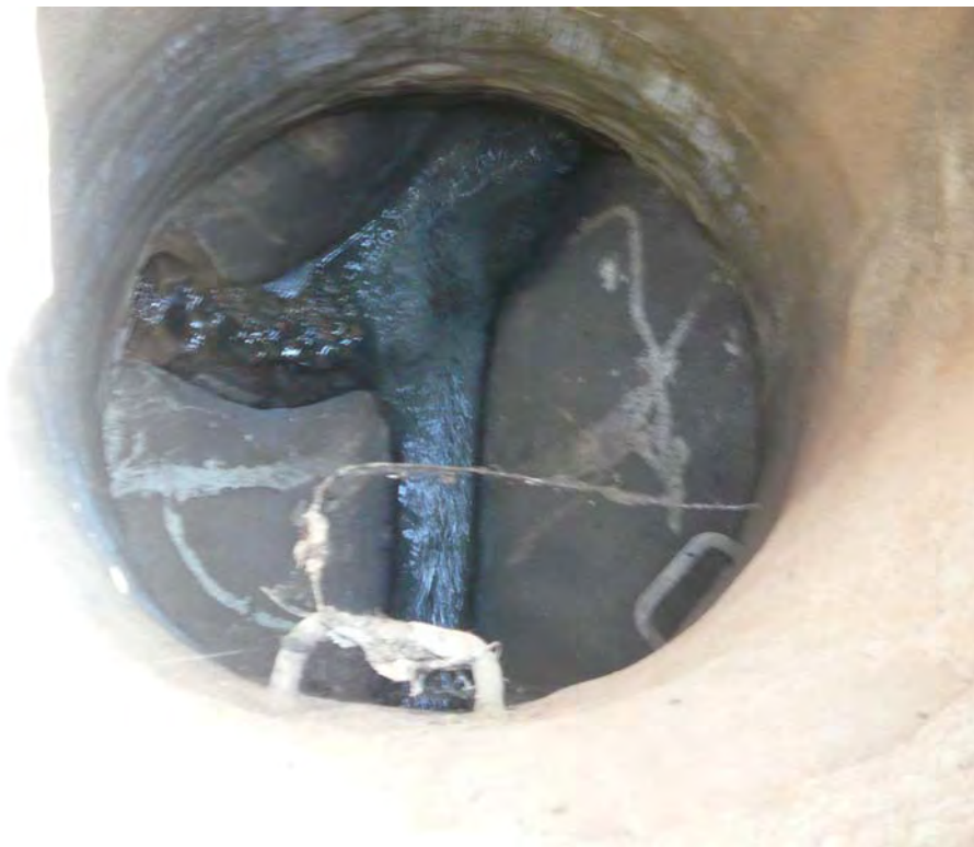
Photo 8 "Stanford & Wellesley" - this is the manhole that now overflows
