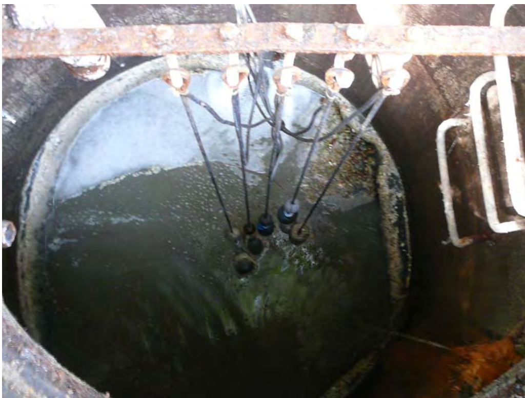
Photo 6 Cannon pump station wet well
