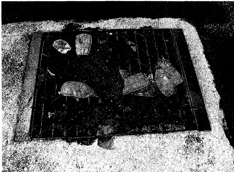
Photo 7 - Close-up of storm drain inlet outside of Horizon Lines maintenance area
