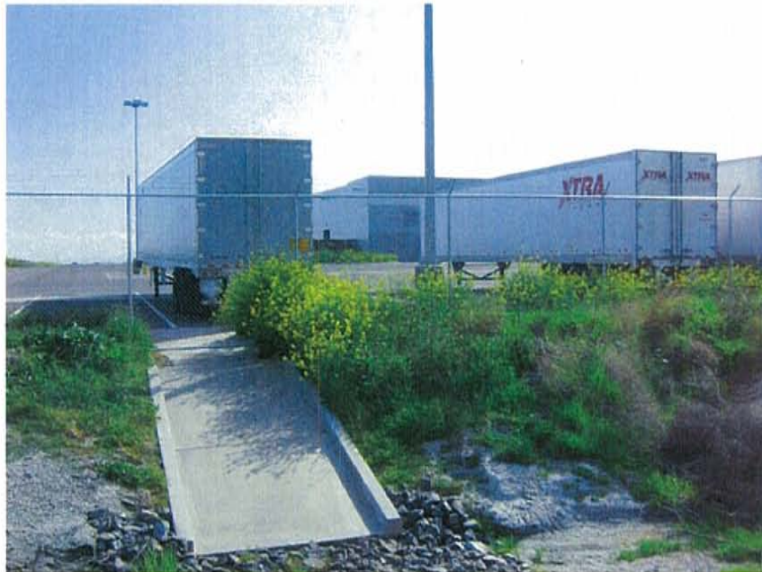
Photograph 16: Newly constructed parking improvements at the Ferguson Distribution Center (looking south).
