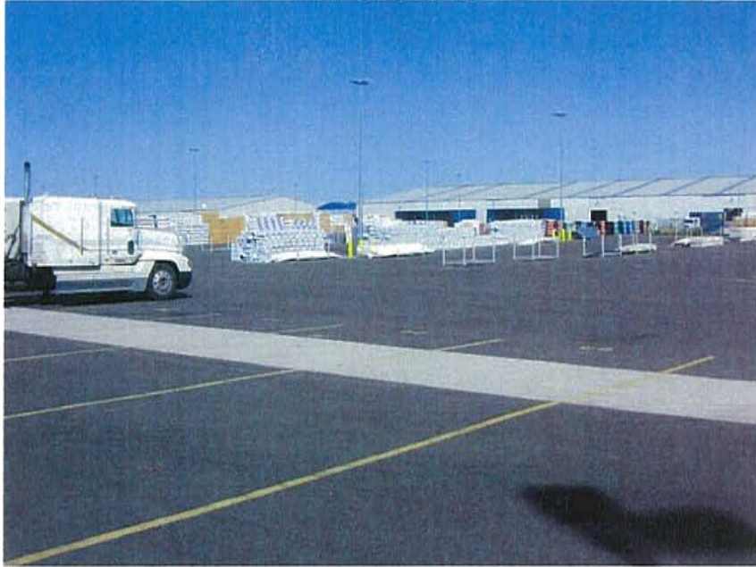
Photograph 13: Impervious parking improvements at the Lowe's Distribution Center (looking north).
