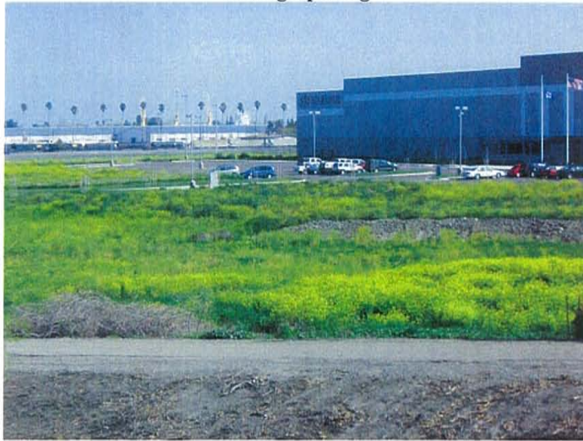
Photograph 15: Newly constructed warehouse structure and impervious parking improvements at the Ferguson Distribution Center (looking east).
