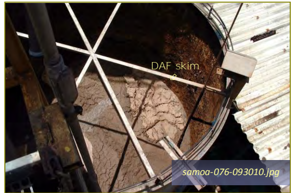
Photo #4: DAF Skim - Holding to High-Strength Tank Taken By: Greg V. Arthur Date: 09/30/10
