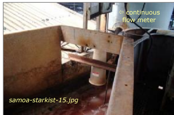
Photo #10: NPDES Sample Point - Flow Meter Taken By: Greg V. Arthur Date: 04/03/08
