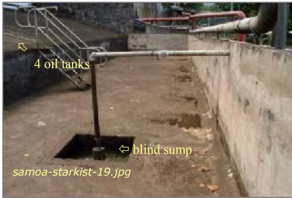
Photo #11: Tank Farm - Showing 2° Containment Taken By: Greg V. Arthur Date: 04/03/08
