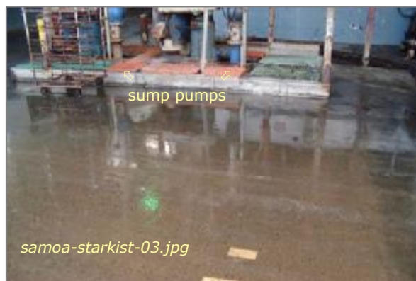
Photo #4: Docksideside Wastewater Sump Taken By: Greg V. Arthur Date: 04/03/08
