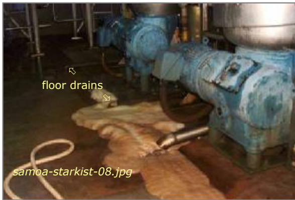
Photo #7: Fish Oil Processing - Decant to Drain Taken By: Greg V. Arthur Date: 04/03/08
