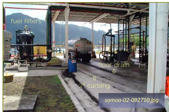
Photo #1-6: Area B - Bottom Fill Loading Rack
