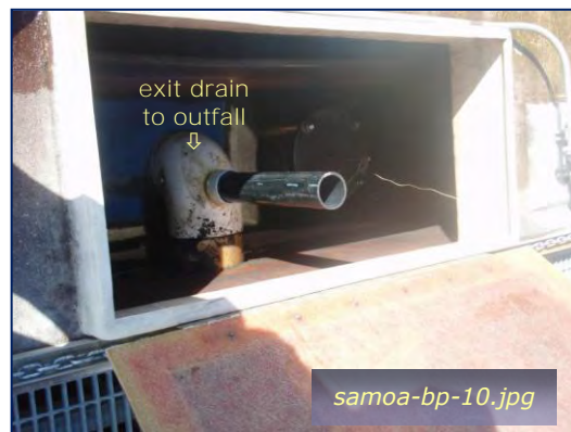
Photo #12: NPDES-003 Discharge Point Taken By: Nick King, Assistant Terminal Manager Date: 06/22/09
