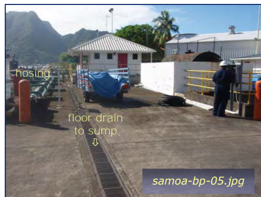
Photo #6: Fueling Dock - looking east Taken By: Nick King, Assistant Terminal Manager Date: 06/22/09
