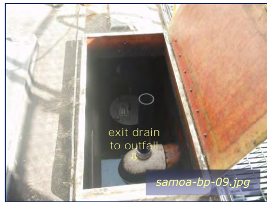
Photo #10: NPDES-002C Discharge Point Taken By: Nick King, Assistant Terminal Manager Date: 06/22/09
