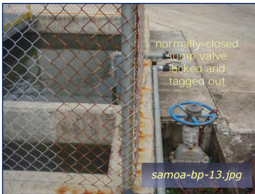
Photo #9: NPDES-002BX Emergency Discharge Point Taken By: Nick King, Assistant Terminal Manager Date: 06/22/09
