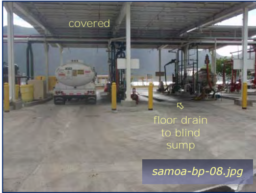
Photo #1: Bottom Fill Loading Rack Taken By: Nick King, Assistant Terminal Manager Date: 06/22/09
