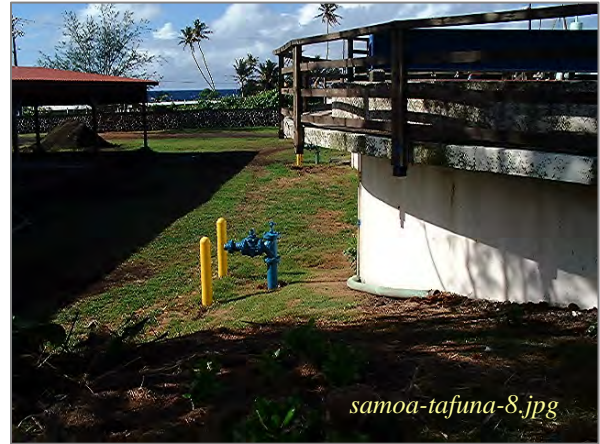
Photo: Tafuna STP – Sludge Draw-off Valving Taken By: Greg V. Arthur Date: 07/16/07
