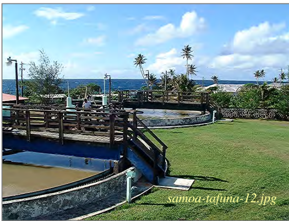
Photo: Tafuna STP – Clarifiers Nos.1 and 2 Taken By: Greg V. Arthur Date: 07/16/07
