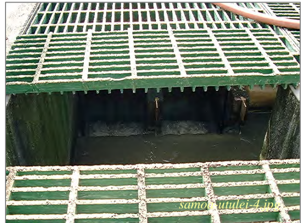
Photo: Utulei STP – Flow Splitter Box Taken By: Greg V. Arthur Date: 07/16/07
