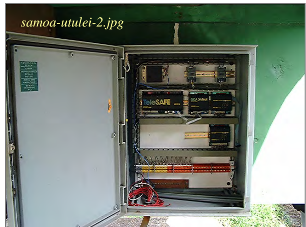
Photo: ASPA Sewers – SCADA Telemetry Taken By: Greg V. Arthur Date: 07/17/07
