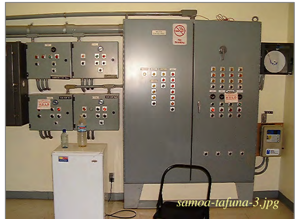
Photo: Tafuna STP – Effluent Monitoring Station Taken By: Greg V. Arthur Date: 07/16/07
