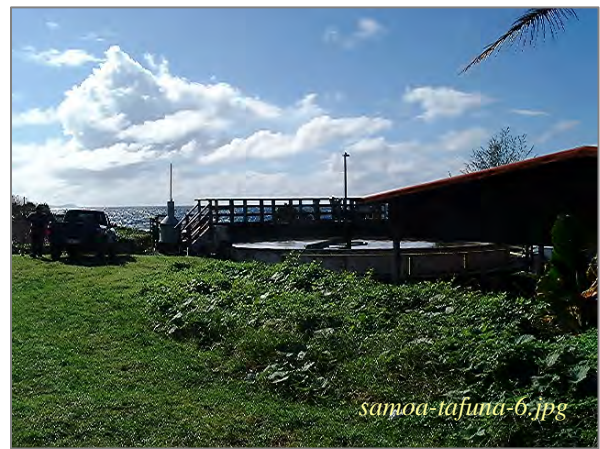
Photo: Tafuna STP – Clarifier No.3 Taken By: Greg V. Arthur Date: 07/16/07
