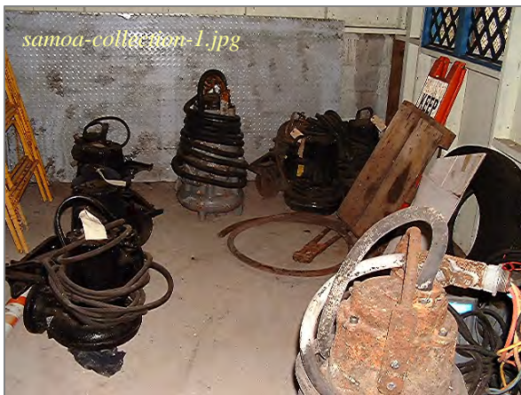
Photo: ASPA Sewers – Stand-by Pumps Taken By: Greg V. Arthur Date: 07/17/07
