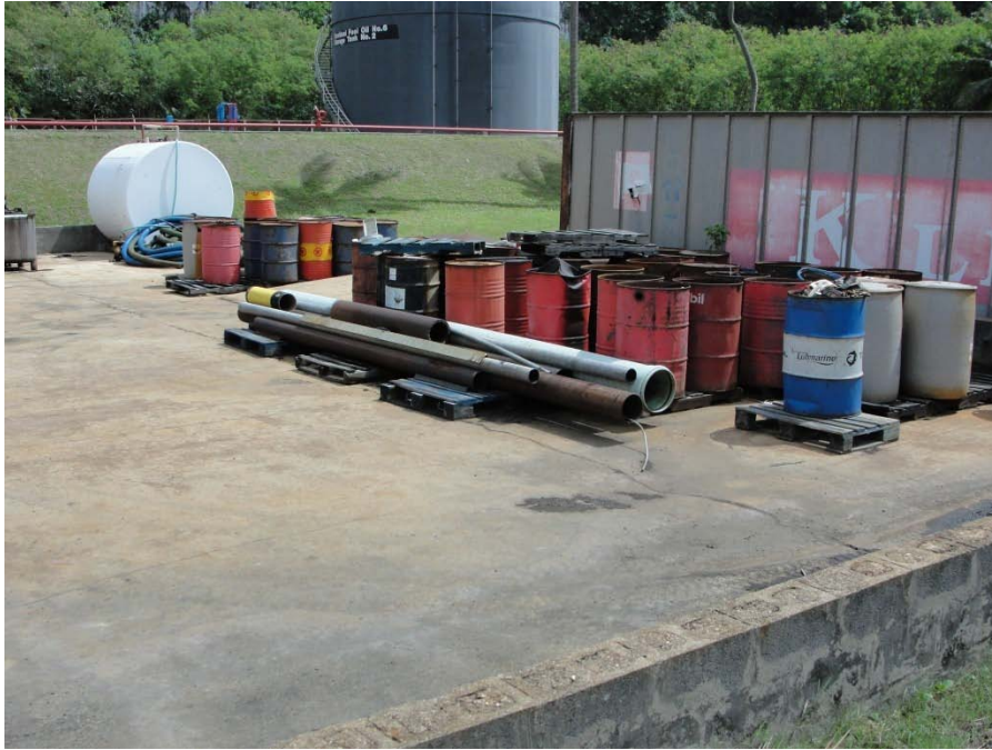
Photo 11: Material storage within secondary containment.
