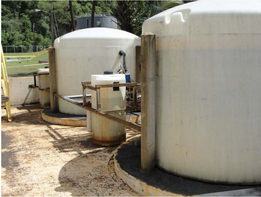
Photo 9: Low volume waste treatment system.
