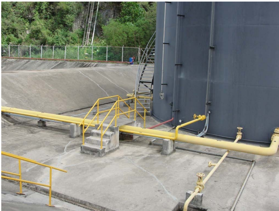
Photo 14: Secondary containment for above ground storage tanks.
