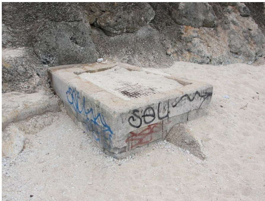
Photo 8: Outfall Serial No. 001B. Note that the outfall is clogged with sand and is not being utilized.
