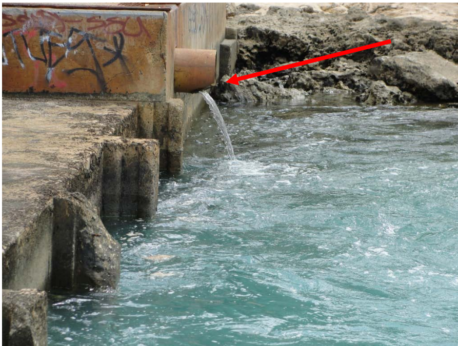
Photo 6: Outfall Serial No. 001A, located adjacent to Outfall Serial No. 001.
