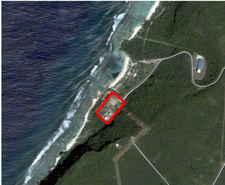
Photo 1: Overview of the Tanguisson Power Plant from Google Maps.
