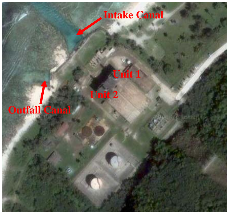
Photo 2: Overview of the Tanguisson Power Plant from Google Maps, with intake canal, outfall canal, and Units 1 and 2 identified.
