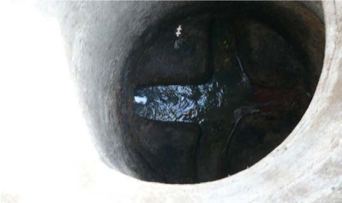
Emeryville Photo 7: Manhole that overflowed at 63rd Street due to debris. Oakland flow enters from left.
