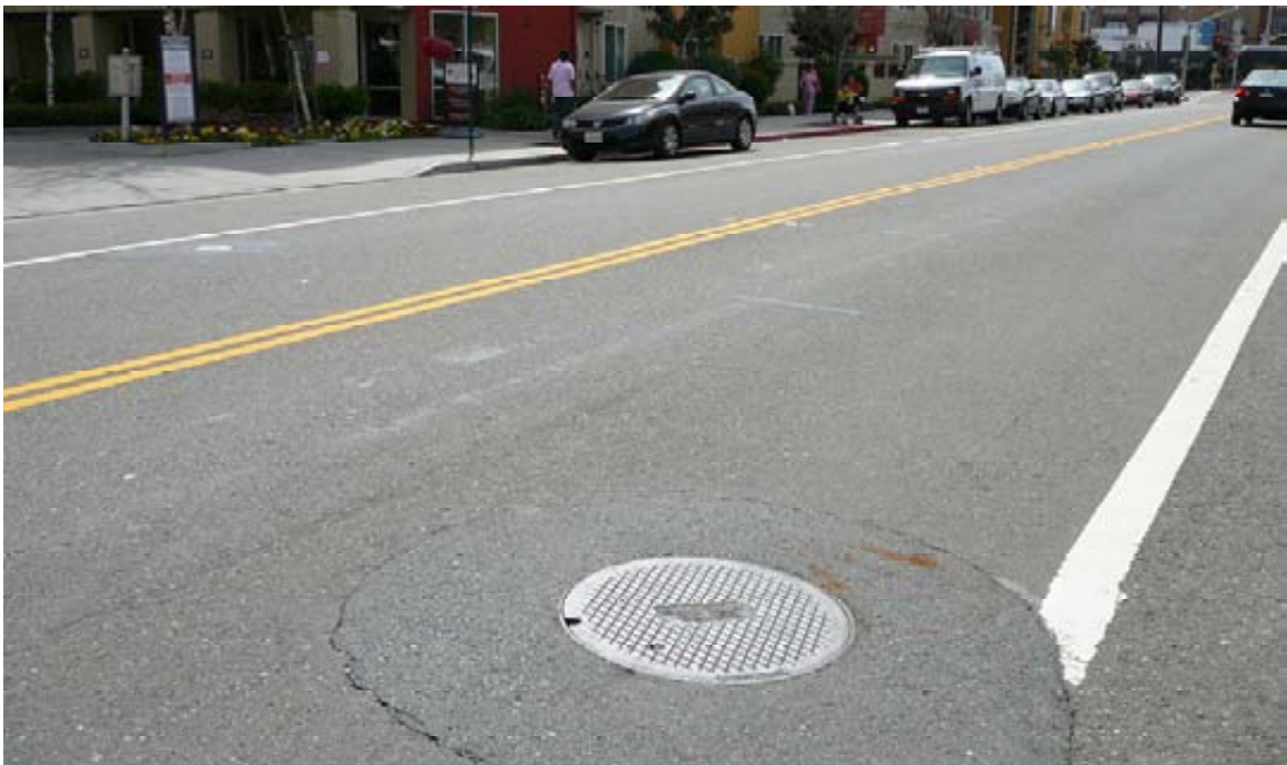
Emeryville Photo 6: 1400 65th Street - manhole cover showing pickhole that wastewater came out of.
