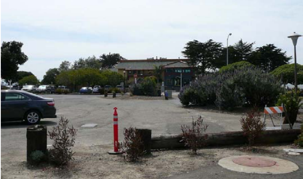
Emeryville Photo 3: View of Hong Kong restaurant from Marina pump station.
