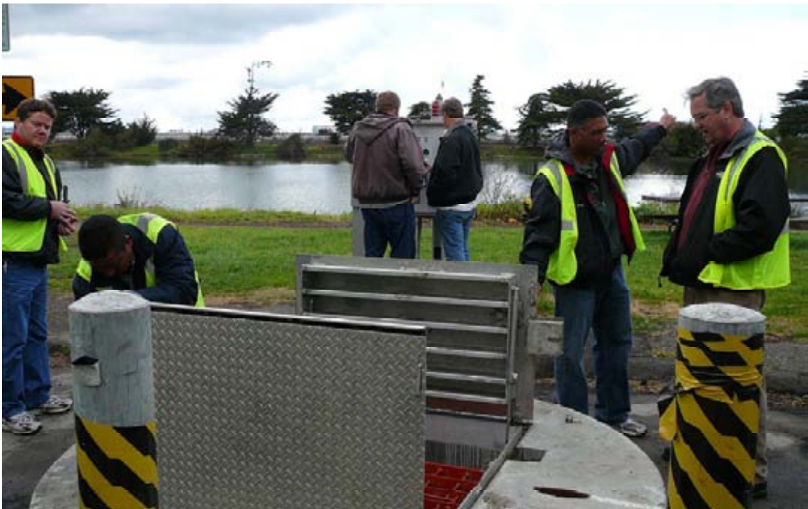
Berkeley Photo 2: Pump station 7 located next to San Francisco Bay.
