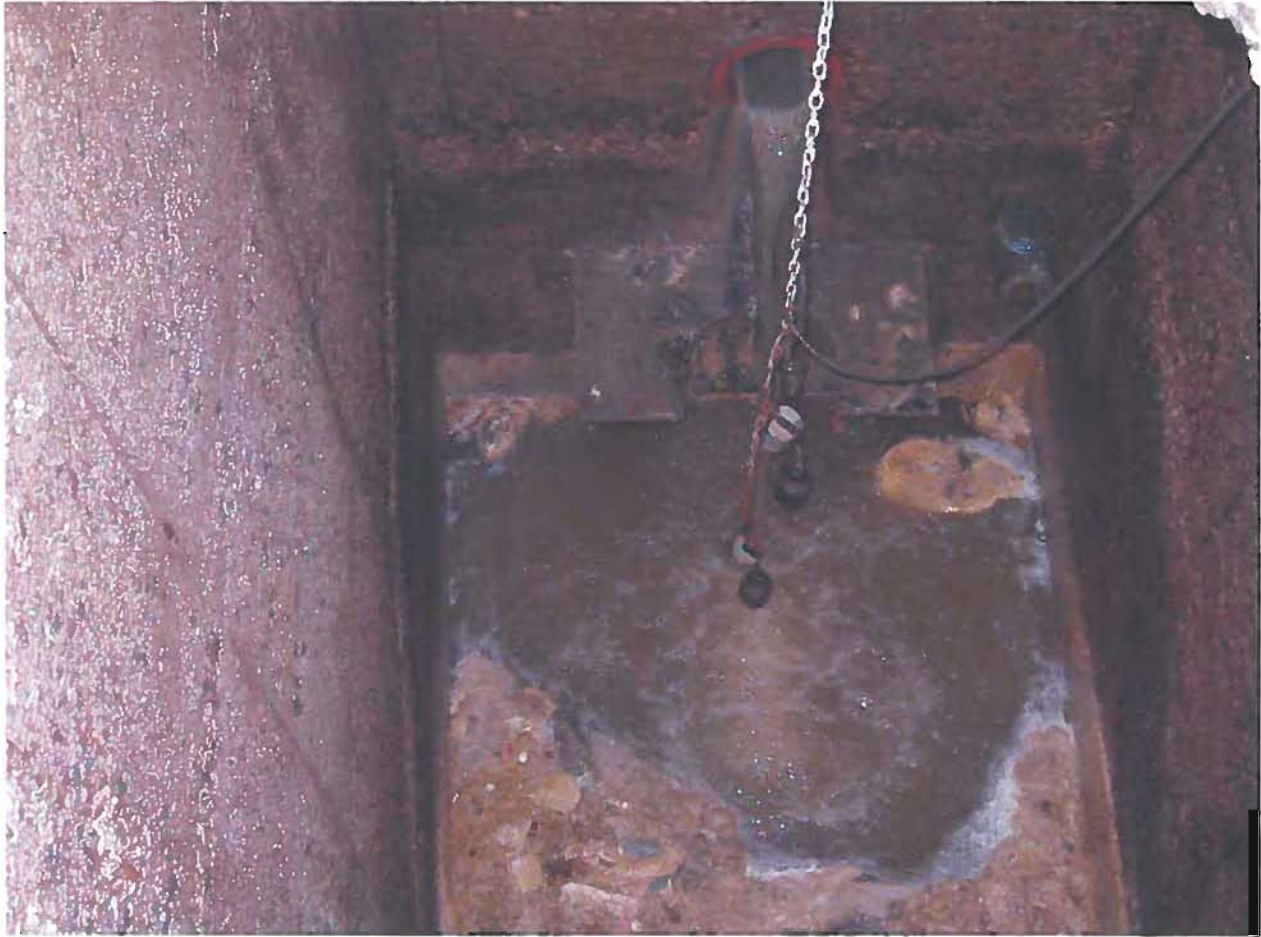
Figure 1: Sewer Plant #7, note the substantial FOG floating on the surface in the wet well. Photograph was taken on December 20, 2011 by Chris Lopez, inspector for the State of California, Los Angeles Regional Water Board.
