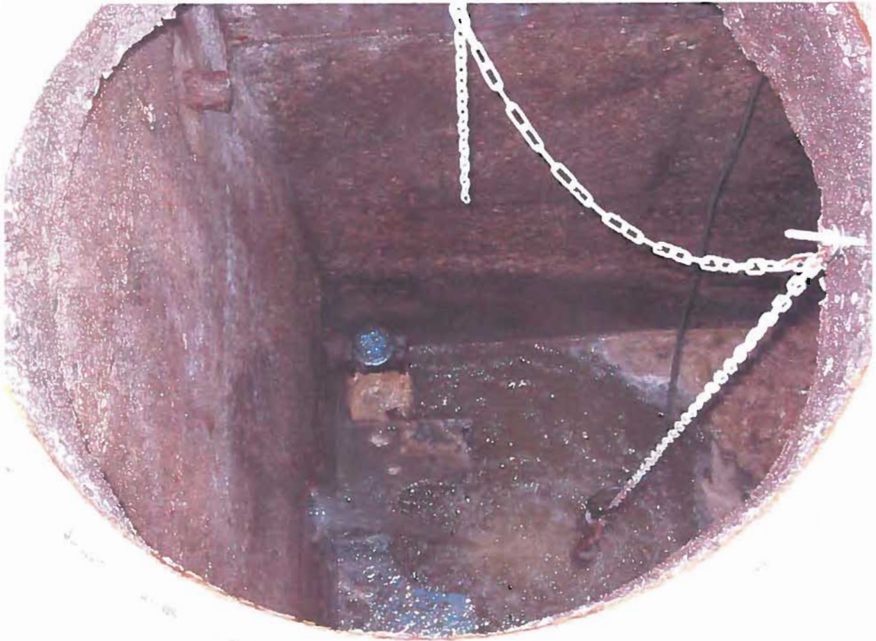
Figure 3: Sewer Plant #7, note the substantial FOG floating on the surface in the wet well. Photograph was taken on December 20, 2011 by Chris Lopez, inspector for the State of California, Los Angeles Regional Water Board.
