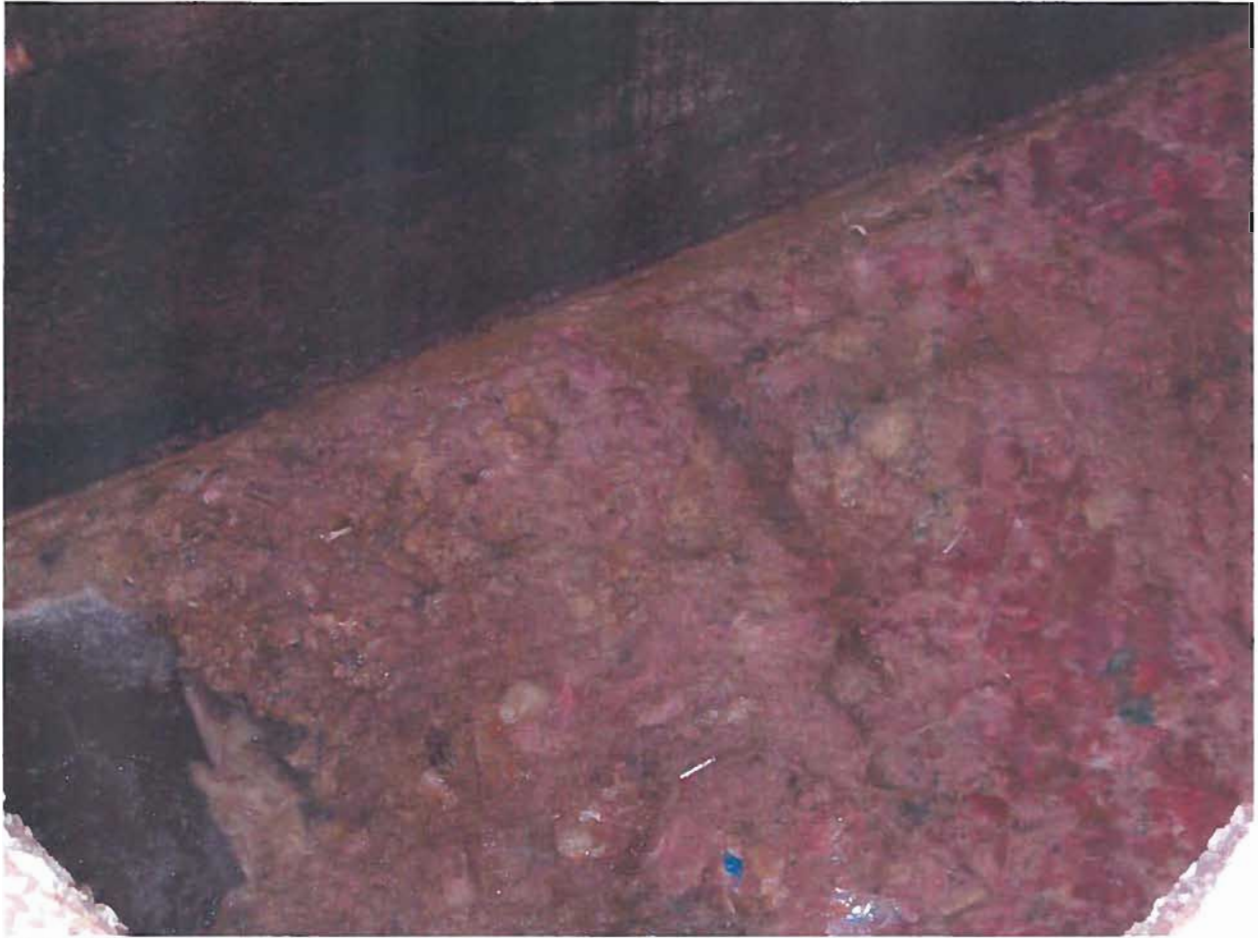
Figure 2: Sewer Plant #7, note the substantial FOG floating on the surface in the wet well. Photograph was taken on December 20, 2011 by Chris Lopez, inspector for the State of California, Los Angeles Regional Water Board.
