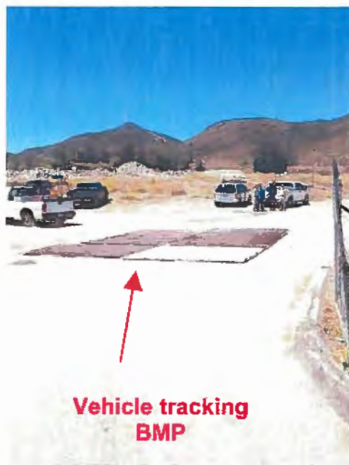
Photograph 1. Wendy Drive/101 Interchange Site Visit – View of a vehicle tracking BMP at the entrance to the material storage area.
