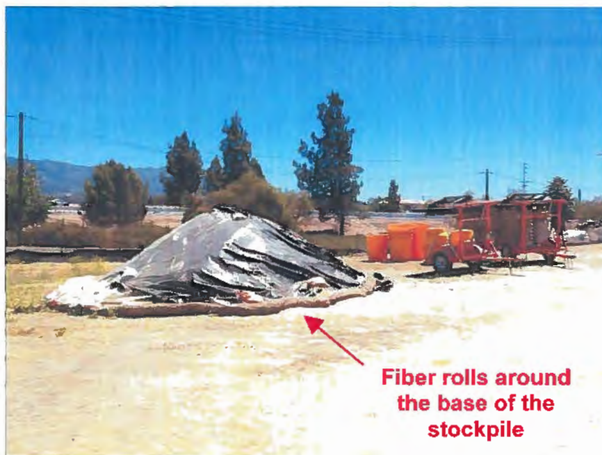
Photograph 2. Wendy Drive/101 Interchange Site Visit – View of material stockpile covered with visquine and fiber rolls at the base of the stockpile.
