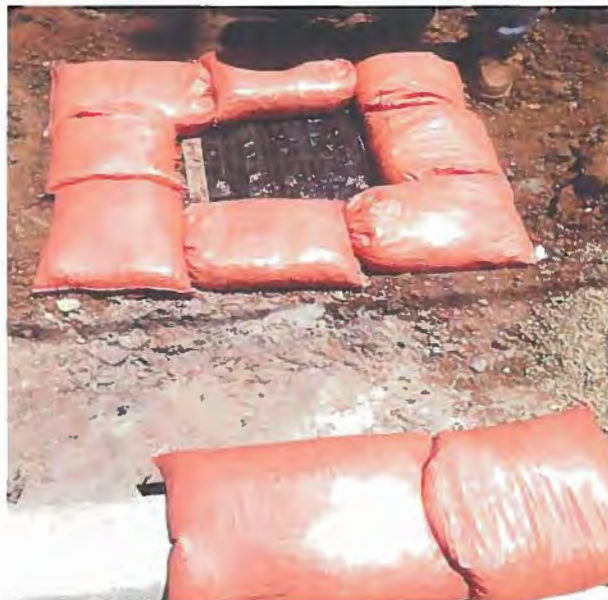
Photograph 9. Many Mansions Site Visit – View of grate inlet covered with geotextile and sand bags placed around the edge of the inlet.
