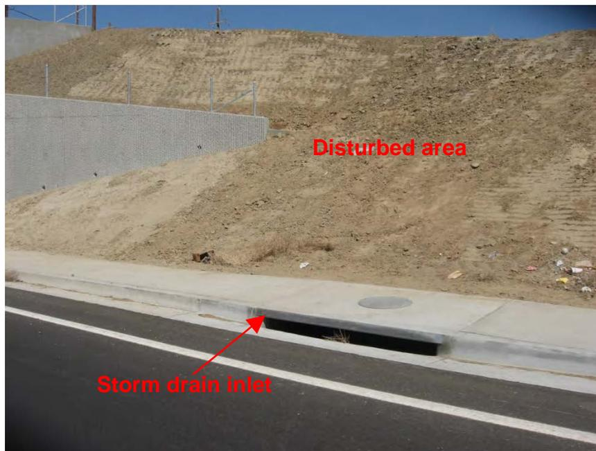
**Photograph 4. View of storm drain inlet without BMPs for inlet protection. Storm drain inlets surrounding the project area were found to be unprotected.**
