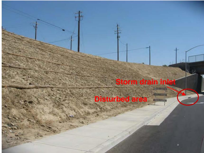
**Photograph 1.** View of wattles which had been installed on several new embankments surrounding the railroad overpass. Note that erosion from the lower level would be discharged to the storm drain inlet because protection had been removed.
