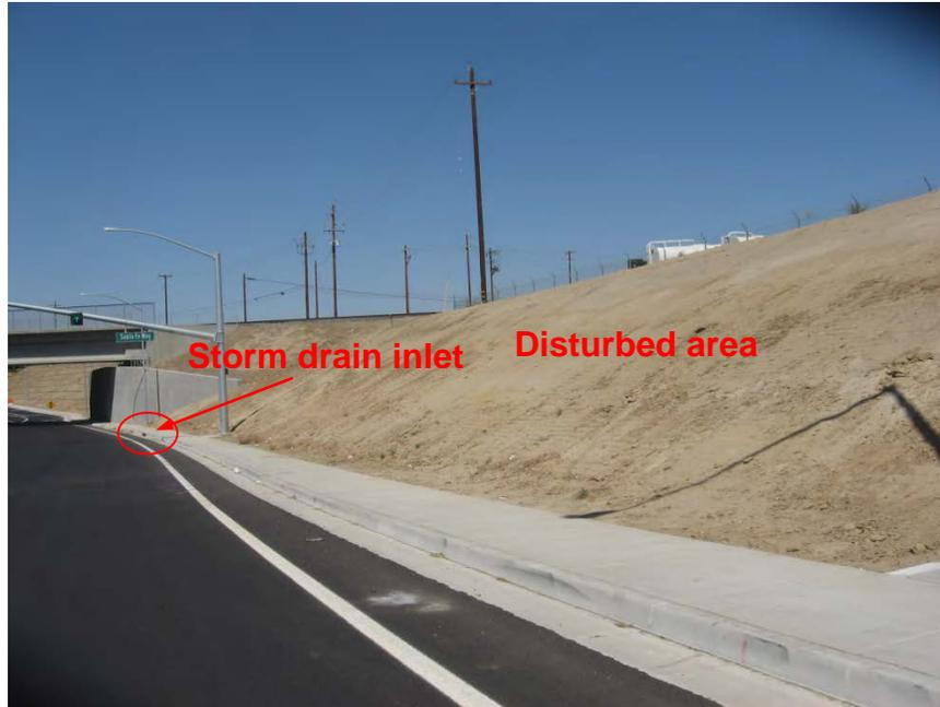
**Photograph 3. View of disturbed slope where wattles were not present on the new embankments south of Hageman Road.**
