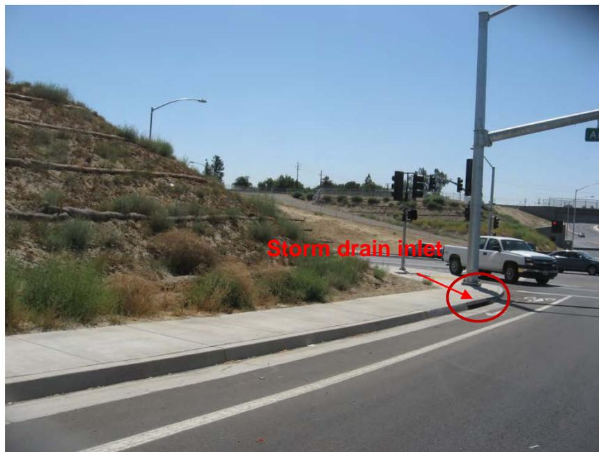
**Photograph 2.** Additional example of wattles which had been installed on several new embankments surrounding the railroad overpass. Note that the storm drain inlet has no protection.
