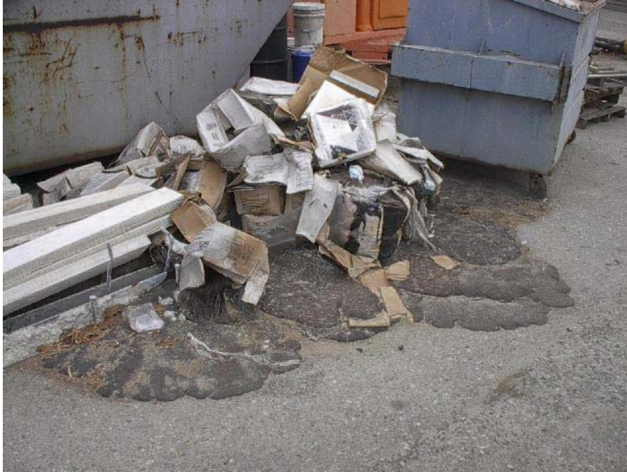
Photo 5: Asphalt patching compound left exposed and now useless. This area drains to the canal, which runs through the yard.
