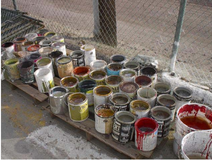
Photo 3: Paint cans left open and exposed. Rain in the past week has filled most of the cans with a mixture of water and paint.
