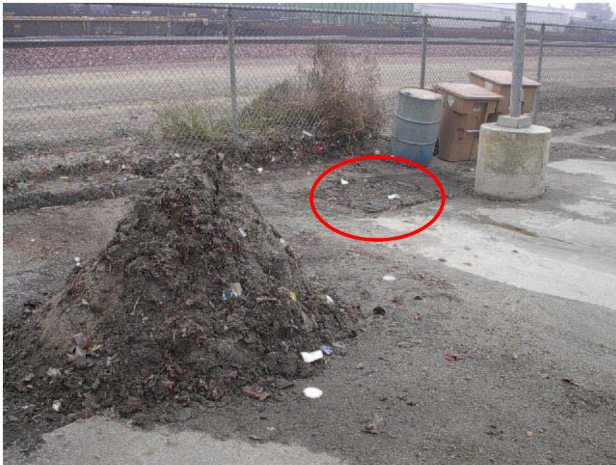
Photo 6: Debris from street sweeper or vactor truck was deposited about 10 feet away from a storm drain inlet (inlet is circled).
