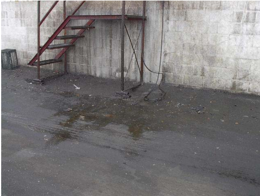
Photo 4: Asphalt cleaning area next to wash rack. Thick layer of asphalt tar on ground. Area discharges to nearby storm drain.
