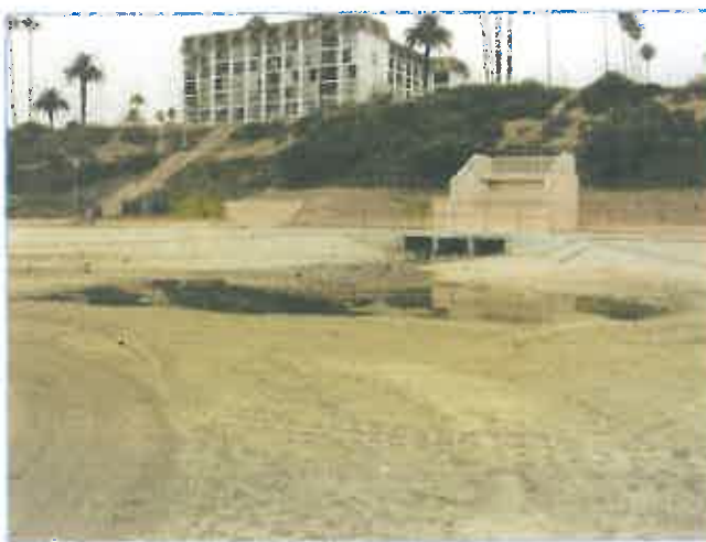
Molino Storm Drain during 2007 dry weather surveys
