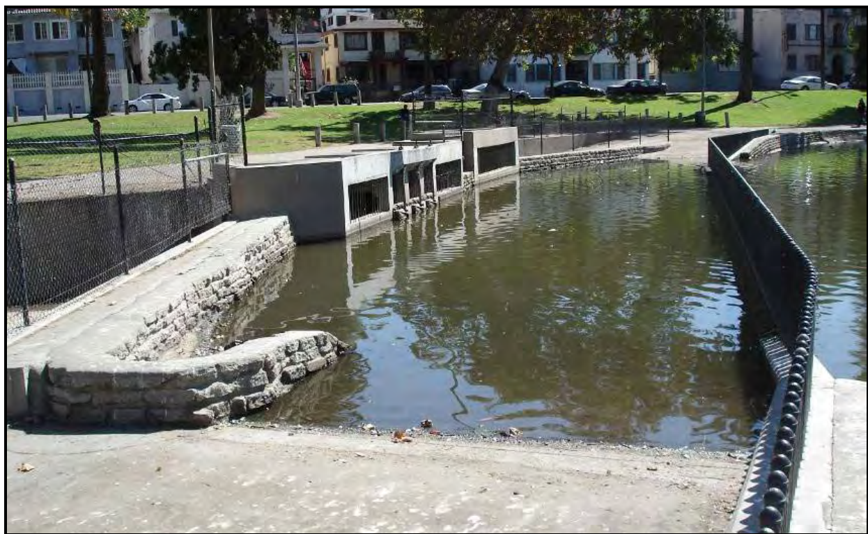
Figure 6-7. Echo Park Lake Northeast Storm Drain Input
